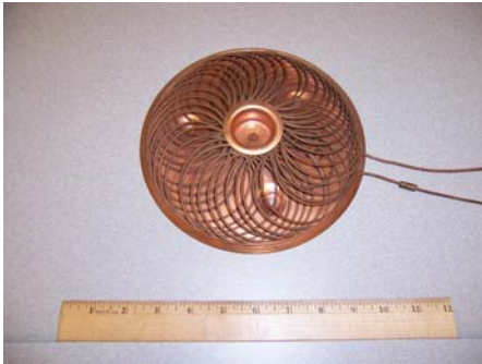
Heat detection device original to building. Removed from M Floor.
