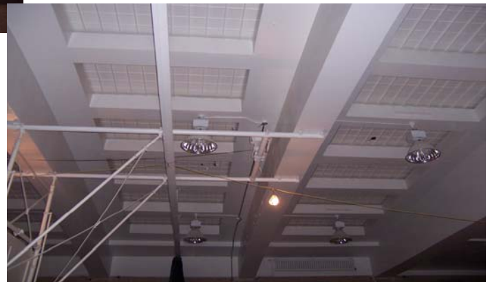
View of roofed over gymnasium skylights
