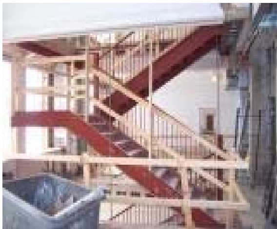
Construction of new stair tower
