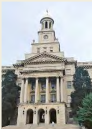
Philadelphia Job Corps Center
