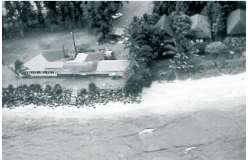
Coastal erosion vs. beach loss. The beach in front of the armored revetment is much narrower than the beach in front of the unarmored segment, where greater shoreline setbacks have allowed more coastal erosion.
