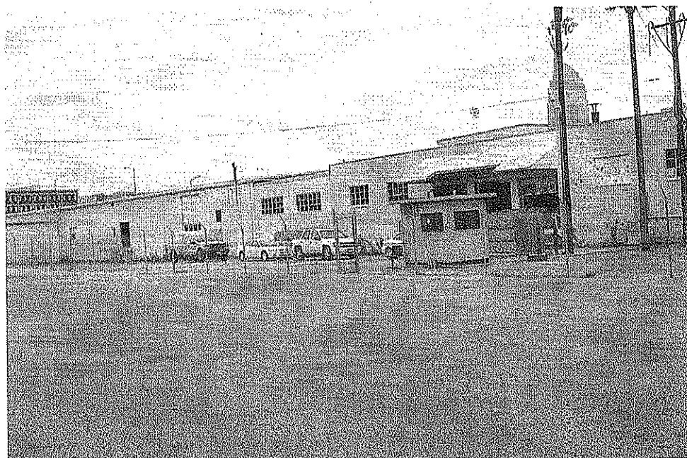
Dico Production Building; view to the east Shows new security fencing and guard shack 9/19/07
