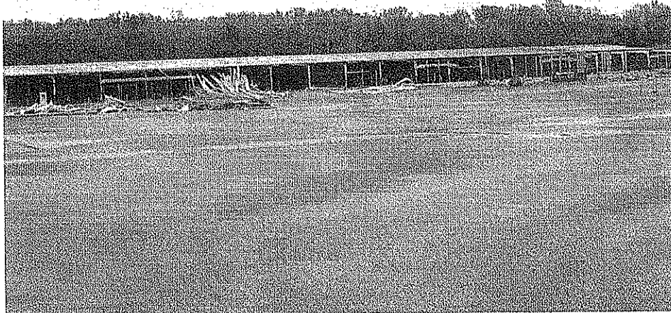
Dico Building 4/5 demolition; view to the east 9/19/07
