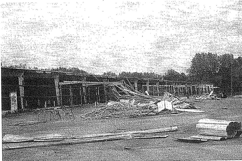
Dico Building 4/5 demolition; view to the south 9/19/07
