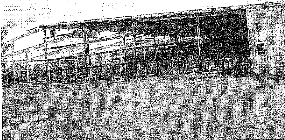
Dico Building 4/5 demolition; view to the northwest 9/19/07
