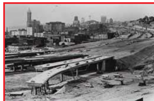
Construction of I-5 through the ID, 1950's, courtesy HistoryLink.org
