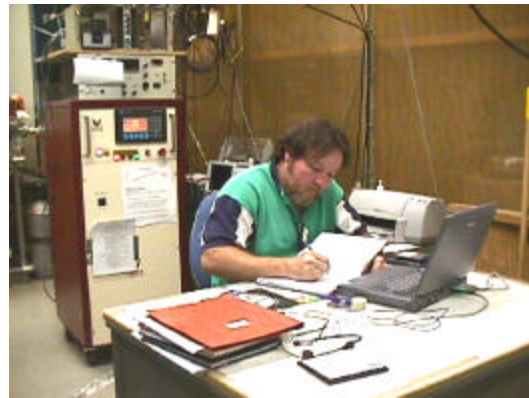
HV AC Power Supply and Partial Discharge Studies
