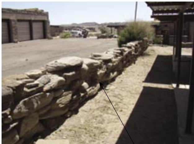
Repair or rebuild historic site walls Photo by author
