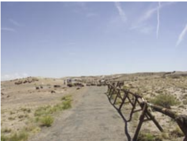
The use of pine pole barricades should be limited to temporary installations. Photo by author
