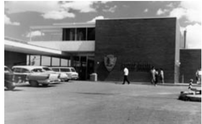
Painted Desert Admin. / Visitor Center shortly after opening in 1963. PEFO Photo Archive #18421
