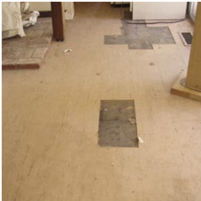
Floor tiles installed prior to 1980 are likely to contain asbestos. Floor tiles are considered non-friable. 2004 Photo by author
