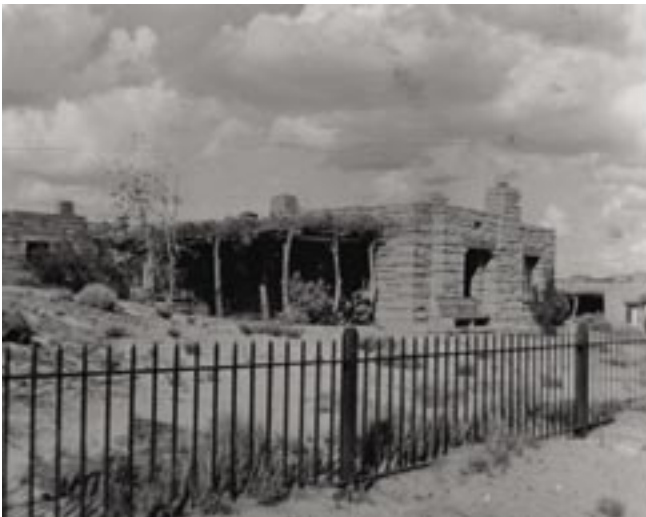
Construction photo of Rainbow Forest buildings showing sandstone masonry construction. PEFO Photo Archive #15867
