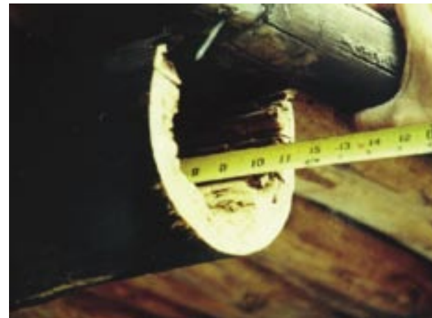
Measuring existing viga for correct diameter and length. Photo courtesy Jake Barrow, NPS
