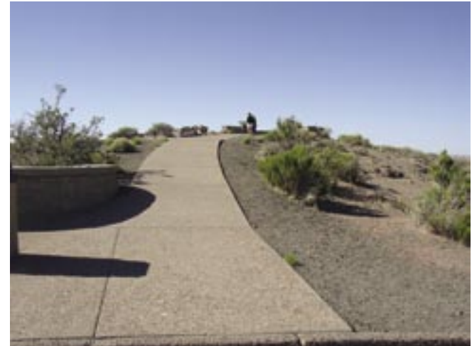
Draining water away from landscape walls and towards parking lots where it can be moved towards the natural landscape is a successful drainage strategy. Photo by author
