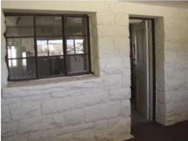
Original 9 pane window at Employee Residence #52-B. Photo by author
