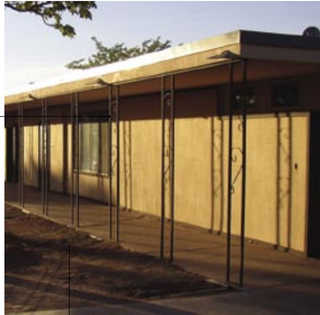
Residence Block B 2004 2004 Photo by author
