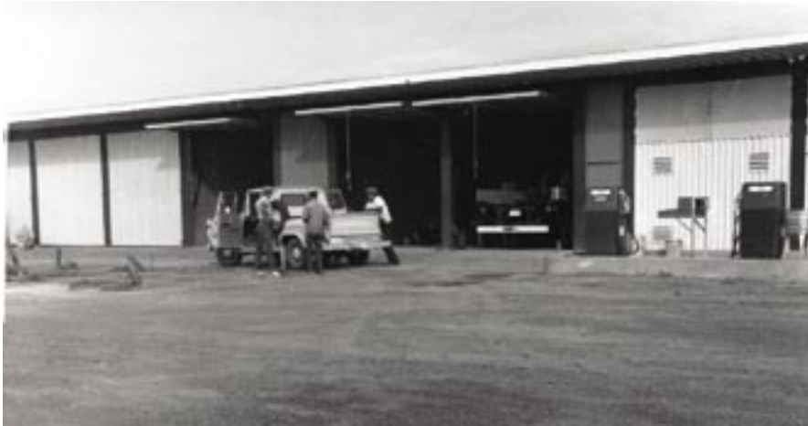
Maintenance building 1963 PEFO Photo Archive 18427
