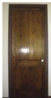
Raised panel door at RF #52-C
