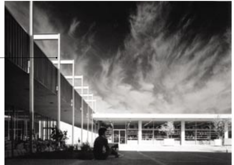
Visitor Center and Fred Harvey Building 1963 PEFO Photo Archives photo by Beinlich
