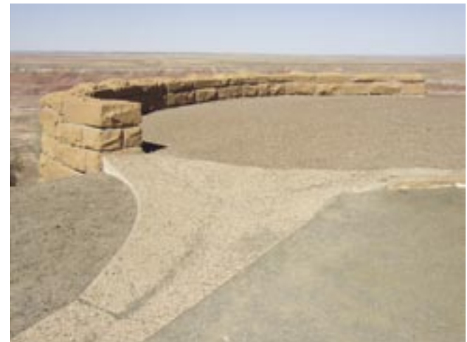
This simple drainage channel at Tawa Point is integrated into the paving material and moves water away from landscape walls. It is also visually pleasing and compliments the color and texture of the wall and paving. Photo by author
