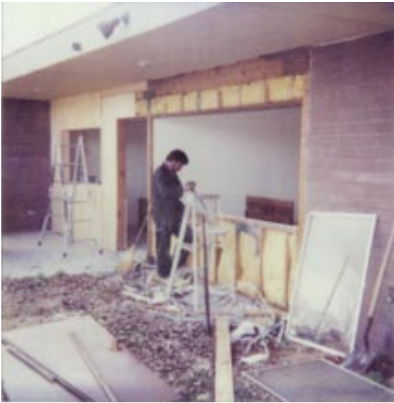
Apartment J undergoing infill c.1980s PEFO Photo Archive, uncataloged
