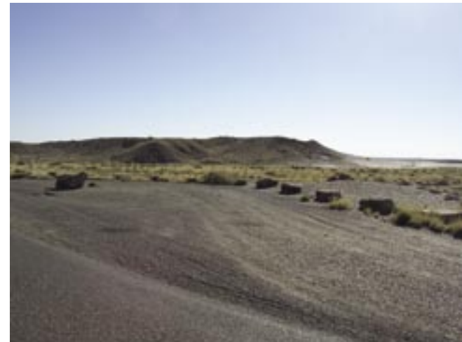
Using large objects, like petrified wood, to keep vehicles from leaving park roads has been used successfully in the park. While the use of petrified wood is no longer possible due to management guidelines restricting its movement the use of boulders may be a possible alternative. Photo by author
