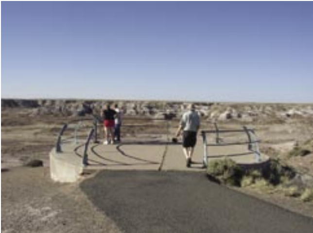
One of the more unusual railings in the park is found at Jasper Forest. Too many different designs could be problematic to repair and maintain. Photo by author
