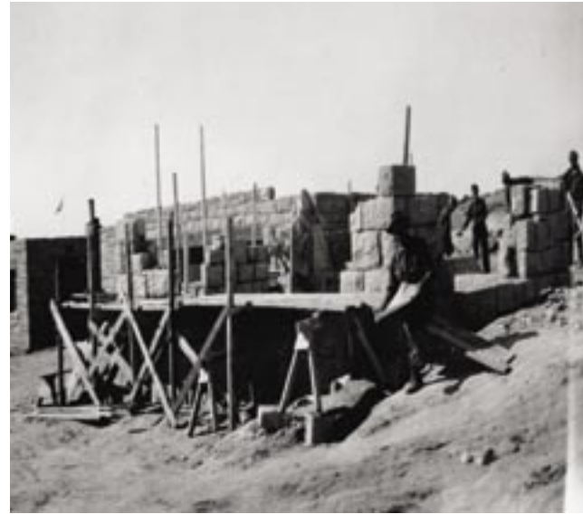
Construction photo of Rainbow Forest buildings showing sandstone masonry construction. PEFO Photo Archive #15867
