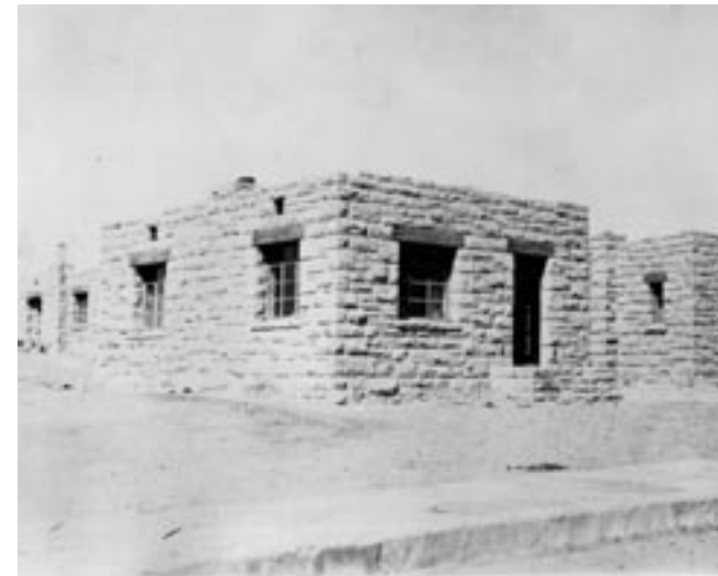
Historic photo of RF52-A showing original 9 lite windows. PEFO Photo Archive #15675
