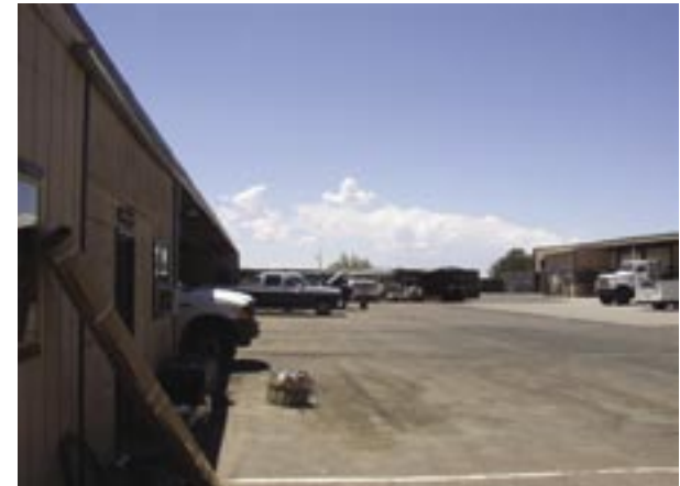
Maintenance and Fire Cache, Vehicle Storage interior yard looking south 2004 Photo by author
