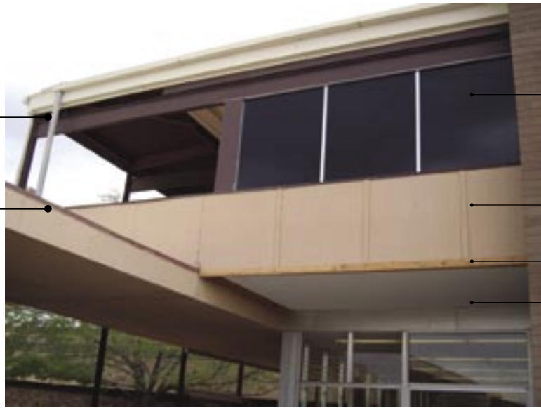
Intersection of PD Oasis and Administration Buildings 2004 Photo by author
