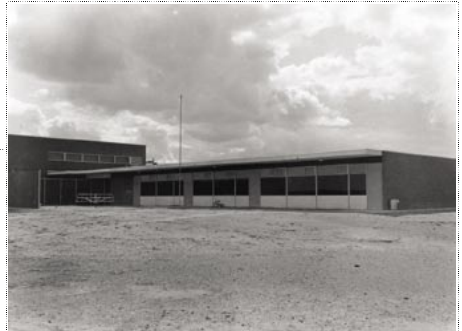
School building east facade c.1965 PEFO Photo Archive photo by Stitt
