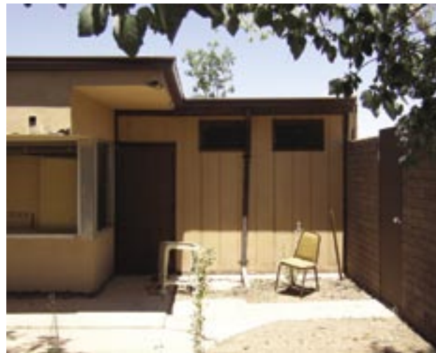
Painted Desert Residential Unit 208. At this scale, it is possible to see how materials come together, like the aluminum windows and roof overhang and the contrast between the smooth stucco walls and brown concrete blocks. Photo by author
