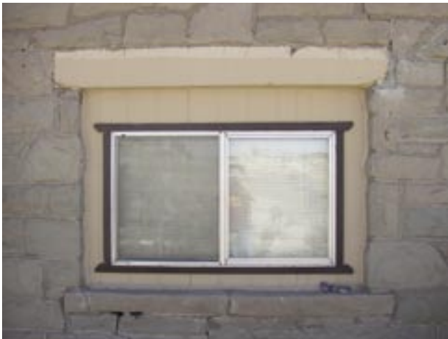
Inappropriate replacement. This aluminum replacement window is too small for the existing masonry opening. Replacement windows shall fill existing masonry openings and infill around windows shall be avoided. Photo by author
