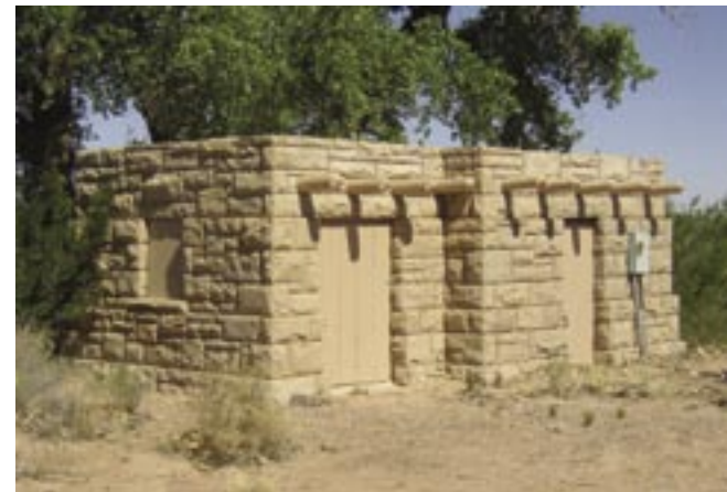
Rio Puerco Pump House, 2004. Photo by author
