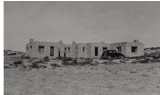
East Elevation of RF Employee Residences 52A, 52B and 52C. Photo date 1938. PEFO Photo Archive #15678
