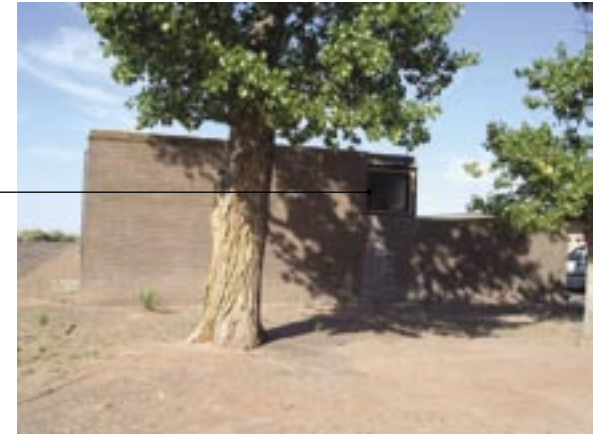
PD 254 north facade 2004 Photo by author
