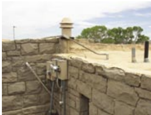
Detail of foam roofing applied to parapet.
