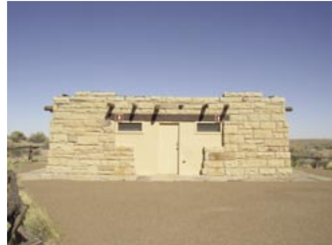
Rio Puerco Comfort Station viewed from the east in 2004.
