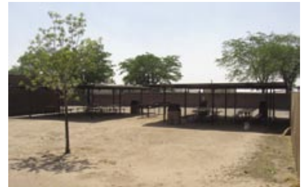
Picnic shelters looking northwest 2004 Photo by author
