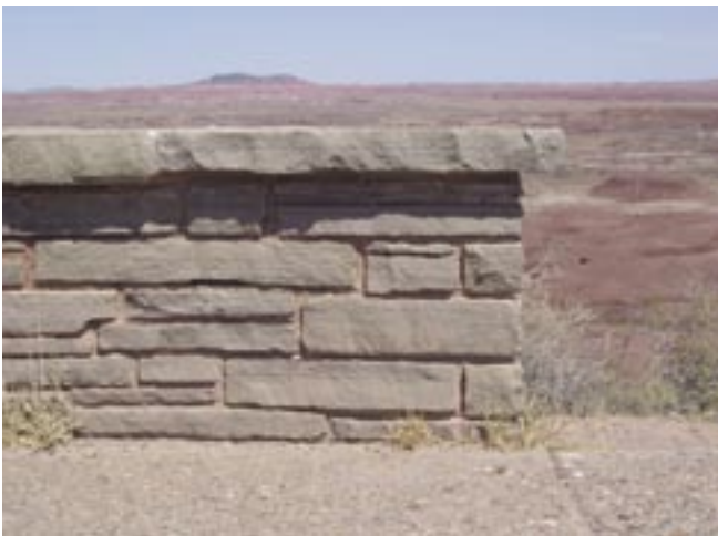
A stone cap provides a distinct shadow line. Photo by author
