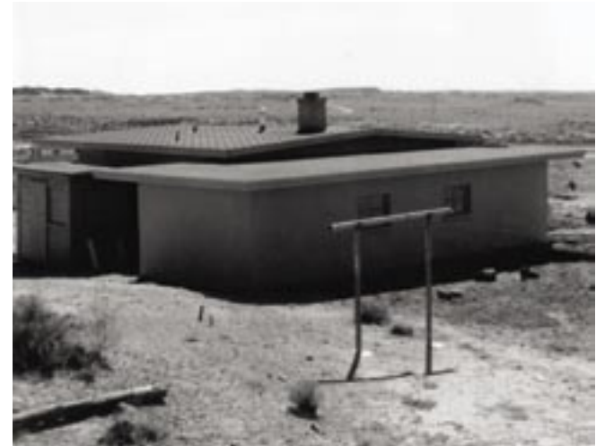
Rainbow Forest Employee Residence #53 looking southeast, 1963. PEFO Photo Archive #23740.11
