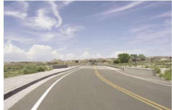
Landscape features built in recent years often overwhelm the natural landscape and lack the natural aesthetic of earlier features. In responding to current transportation regulations that require wider lanes, the Jim Camp Wash Bridge completed in 2002, became a more significant element in the landscape. Also, of note, is the use of monolithic concrete walls that lack the texture and color of earlier features found in the adjacent Rainbow Forest Historic District. Photo by author
