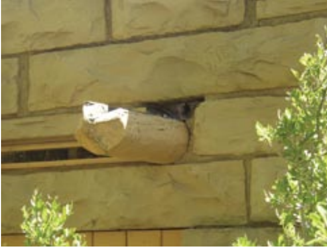
Existing viga end, with integrated canales, at Rio Puerco Comfort Station. Photo by author
