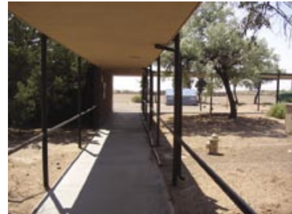
Covered walkway looking east 2004 Photo by author
