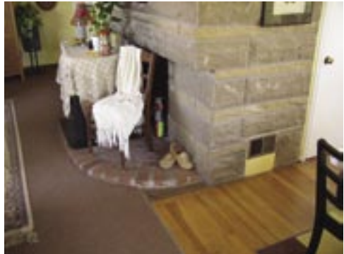
Employee Residence #50 has many of its original historic furnishings intact, including wood flooring and an unpainted sandstone masonry fireplace. The brick hearth and carpet have been added. Photo by author.
