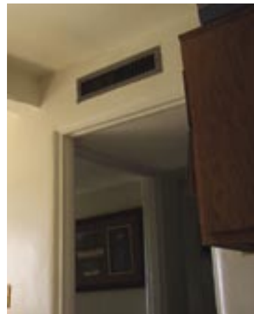
Typical interior door frame at RF residential units. Photo by author
