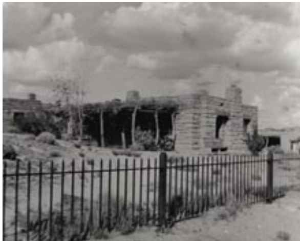
Historic wrought iron fencing with Unit #51-A in background. PEFO Photo Archive #15693
