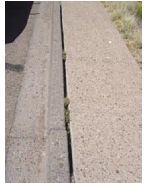
Exposed aggregate curb and gutter at Whipple Point. Note how use of exposed aggregate concrete for the curb relates to the adjacent walk. Photo by author
