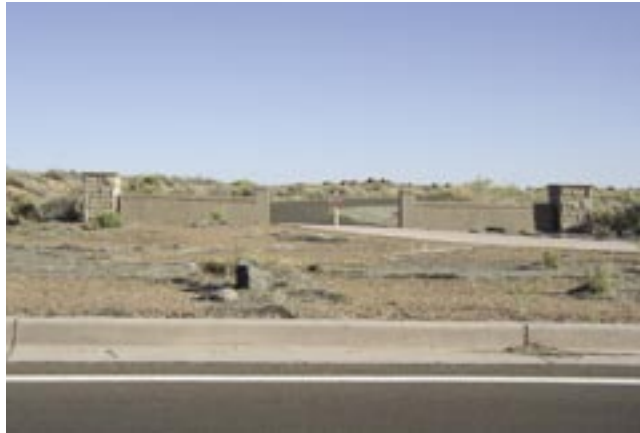
The entrance to the Long Logs trail head reveals the challenge of modifying existing landscape elements. The addition of unadorned concrete walls contrasts sharply with the older stone piers that remain from the entrance to a vehicular road since abandoned. While the use of concrete in this situation is not an unworkable solution, it does illustrate the need for more careful consideration of its visual qualities and how they react with more rustic materials. Photo by author
