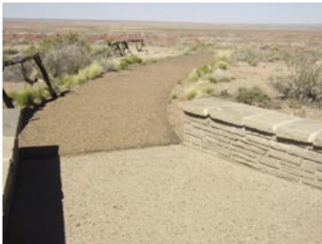
A smooth transition at a change in materials. In this example from Tawa Point, the edge of the exposed aggregate concrete walk aligns with the end of the low wall. Photo by author
