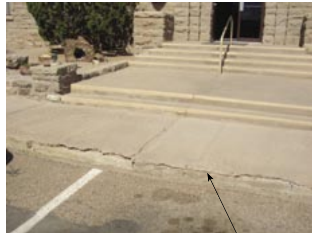
Repair concrete walks and sandstone curbs Photo by author
