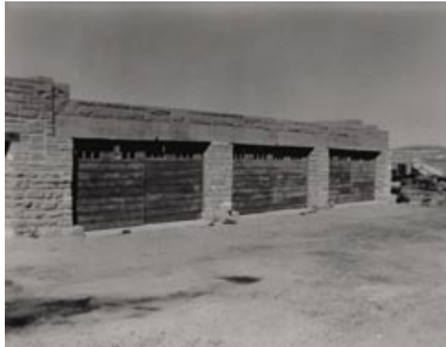
South Elevation of Rainbow Forest Garage, 51E from 1949. PEFO Photo Archive #15701
