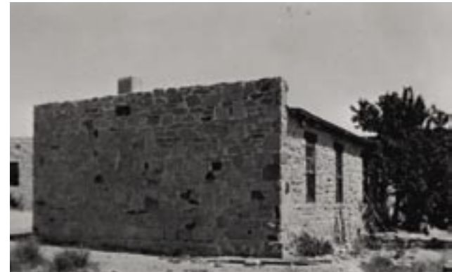
Rainbow Forest Cabins, looking north 1949. Note flat roof with parapets. PEFO Photo Archive #15743
