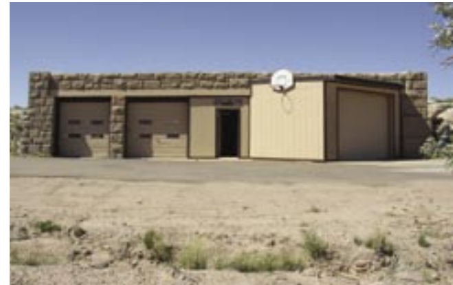
Rainbow Forest Warehouse and Shop with V-Shaped addition, 2004. Photo by author
