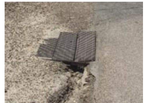
Tripping hazards, such as this drainage grate, should be properly maintained. Photo by author
