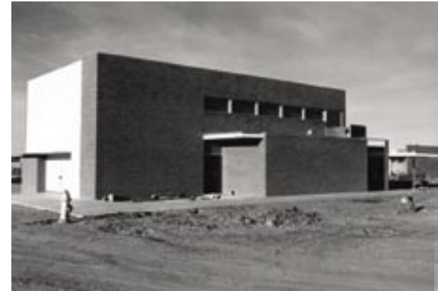
Community building c.1963 notice clerestory windows PEFO Photo Archive Photo by Stitt
