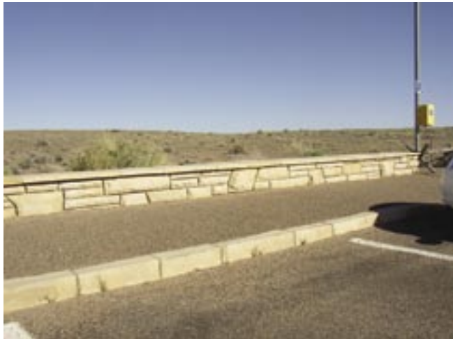
Stonework was used for the curbs and landscape walls at early park landscape features, such as the area around Puerco Pueblo, shown above. Photo by author
