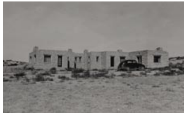
Rainbow Forest #52A-C viewed from the east. Note the texture of the rough faced stone used to construct walls and the smaller projections used to break up the building mass. PEFO Photo Archive #15678
