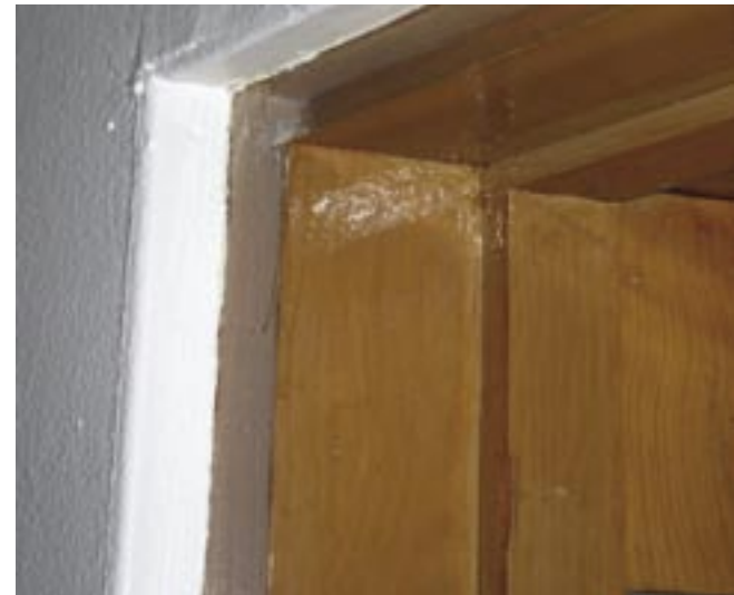
Painted Desert Community Complex detail at interior door jamb. This detail shows the how interior door jamb's are recessed from the drywall surface of interior walls. It also shows Neutra's attention to how a frame is constructed and how his use of materials created a very light and natural feeling on the interior. Photo by author
