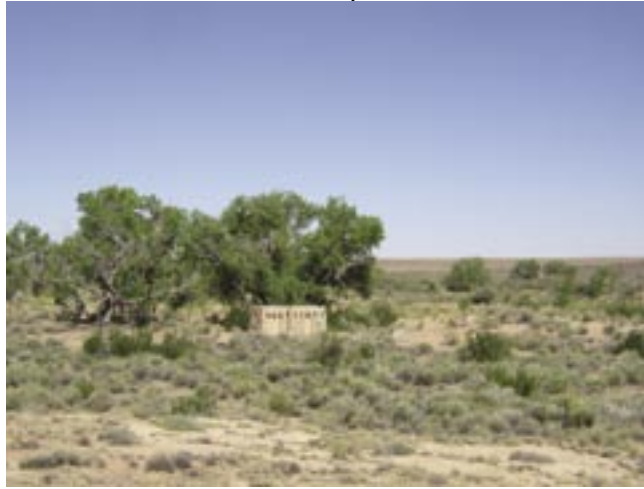
Puerco pumphouse is placed away from major viewsheds. Photo by author
