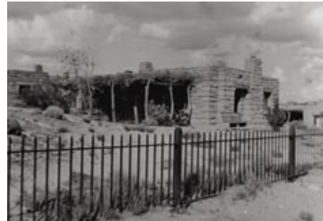
Rainbow Forest Employee Residence #51A with attached wood pole ramada. Photo date 1949. PEFO Photo Archive #15693
