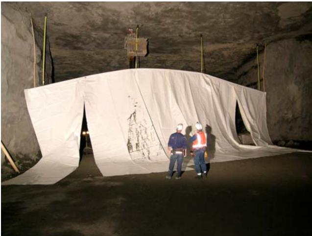
Figure 6. Raising the EZ-Up Curtain Stopping into position.
