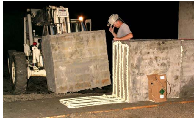
Figure 3. Placing Supper Stopping block in place after applying adhesive.
