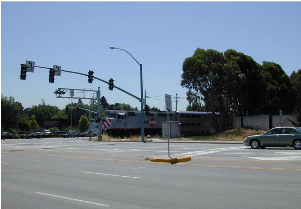
Figure 51. Pre-Signal Located Ahead of Grade Crossing with Displaced Stop Bar, S. Mary and W. Evelyn at Caltrain Commuter Line, Sunnyvale, California
