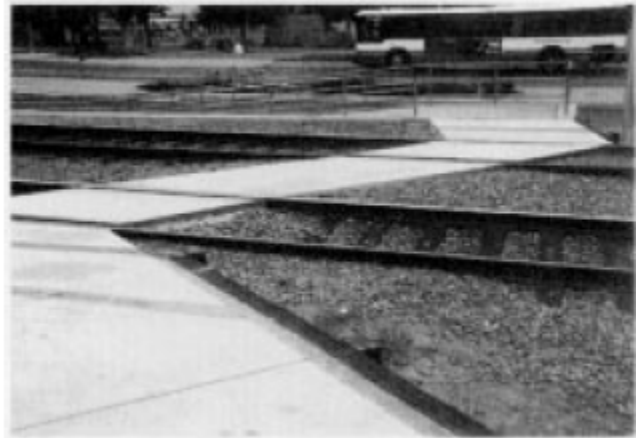
Figure 79. San Diego, California Pedestrian Z-Crossing
