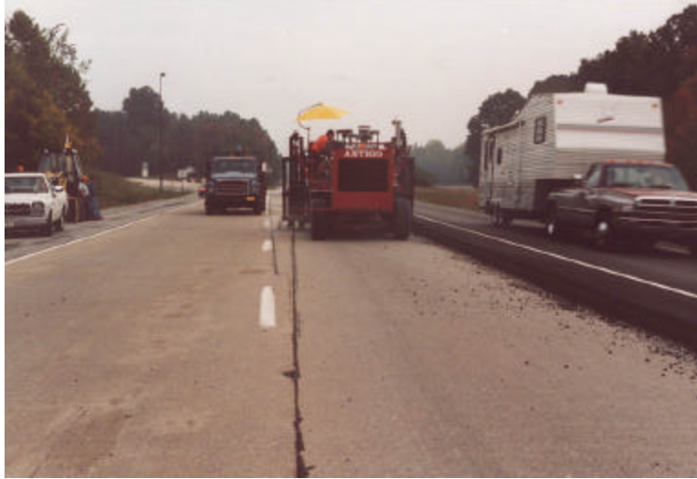
Figure 30. Passing Lane Binder, Driving Lane Rubblizing Begun (I-57 1997).
