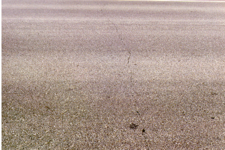
Figure 13. Rubblize and Overlay in 1996 (IL 38 1994).
