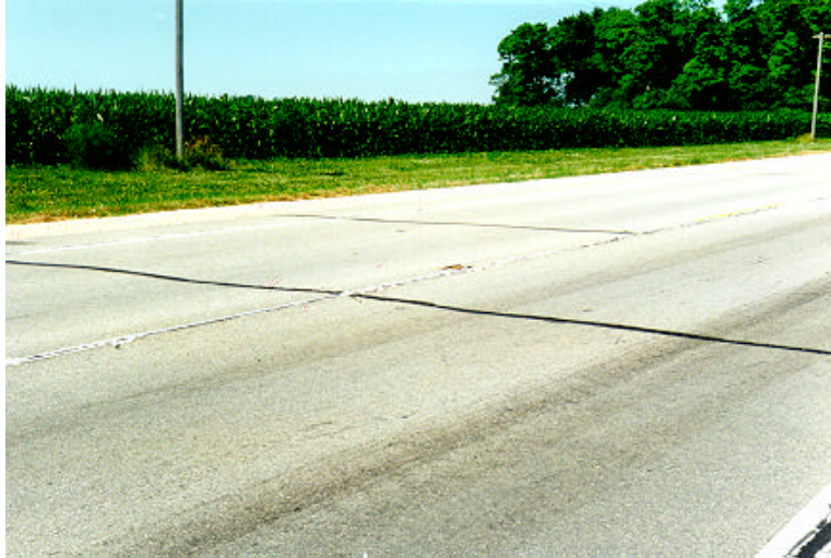
Figure 14. OGBC and Overlay in 1997 (IL 38 1994).
