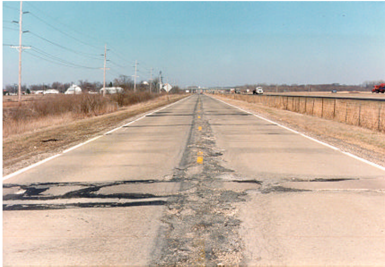
Figure 17. Preconstruction Condition (I-55 FR 1994).
