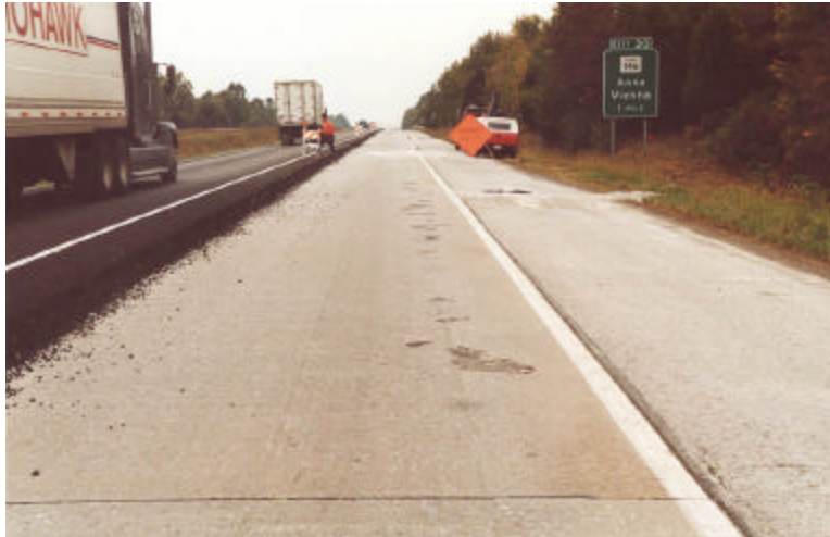
Figure 29. Preconstruction Condition (I-57 1997).
