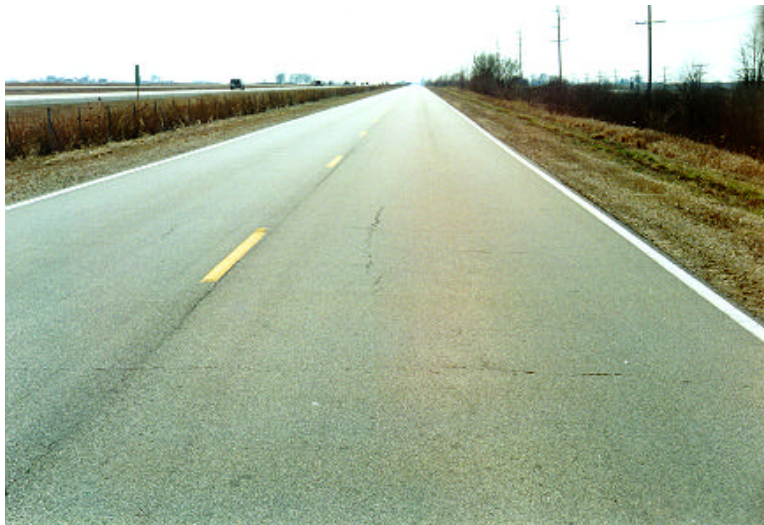
Figure 19. Rubblized/Overlaid Pavement in 1997 (I-55 FR 1994).
