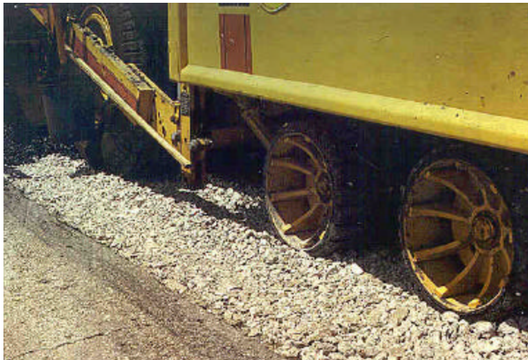
Figure 23. Rubblized Material Moving Under Bogey Tires of Paver (I-57 1996).
