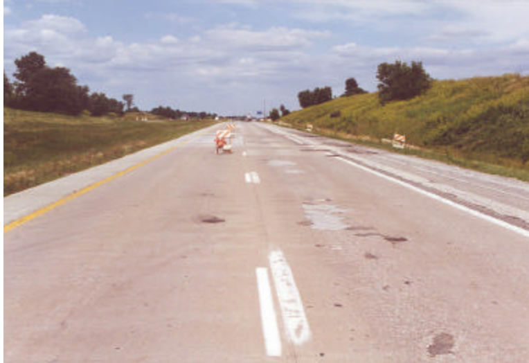
Figure 32. Preconstruction Condition (I-74 1999).
