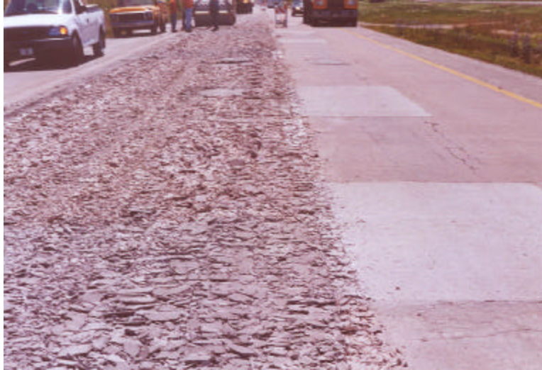
Figure 33. Driving Lane Rubblization (I-74 1999).
