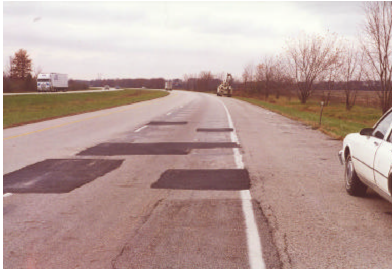
Figure 26. Preconstruction Condition (I-70 1997).
