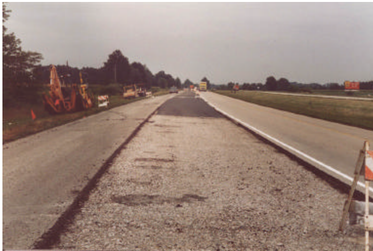
Figure 27. Driving Lane Rubblized and One Lift Binder (I-70 1997).
