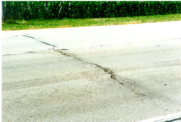
Figure 15. Control Section in 1997 (IL 38 1994).
