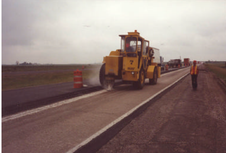
Figure 6. Passing Lane Binder Complete, Driving Lane Begun (I-57 1990).
