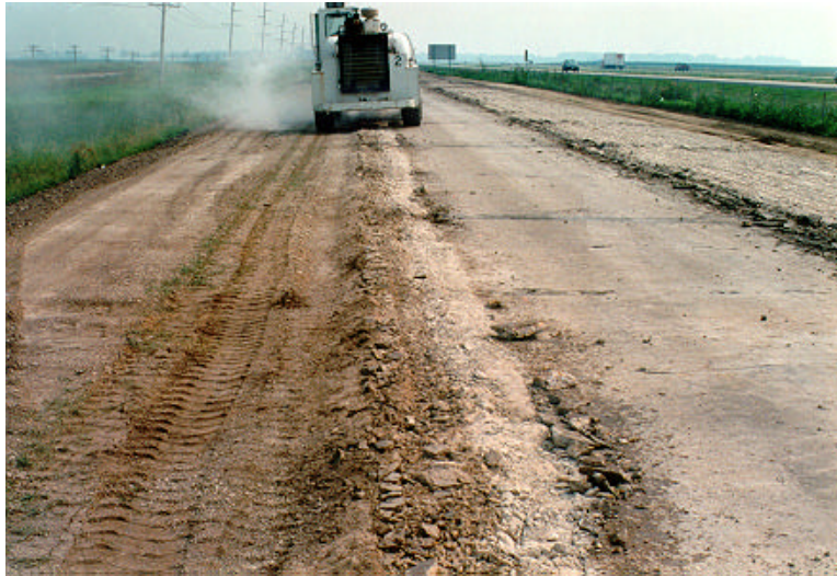
Figure 18. Rubblizing Process (I-55 FR 1994).
