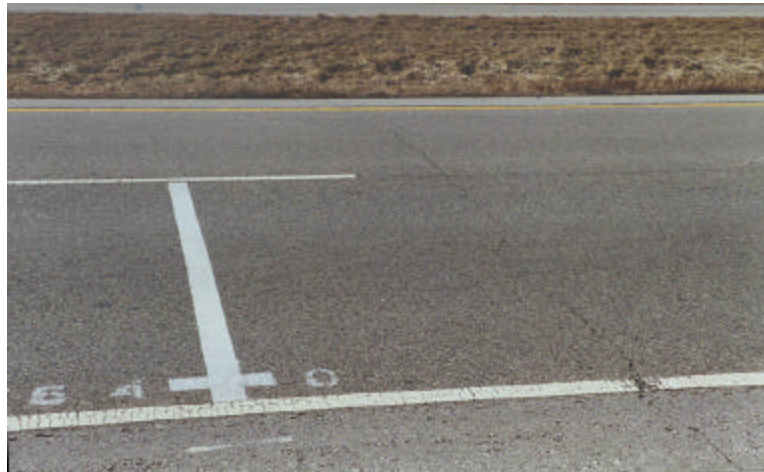
Figure 7. Rubblize and 6" Overlay in 1996 (I-57 1990).
