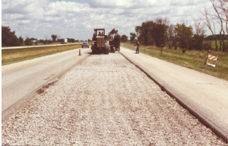
Figure 22. Driving Lane Rubblizing (I-57 1996).
