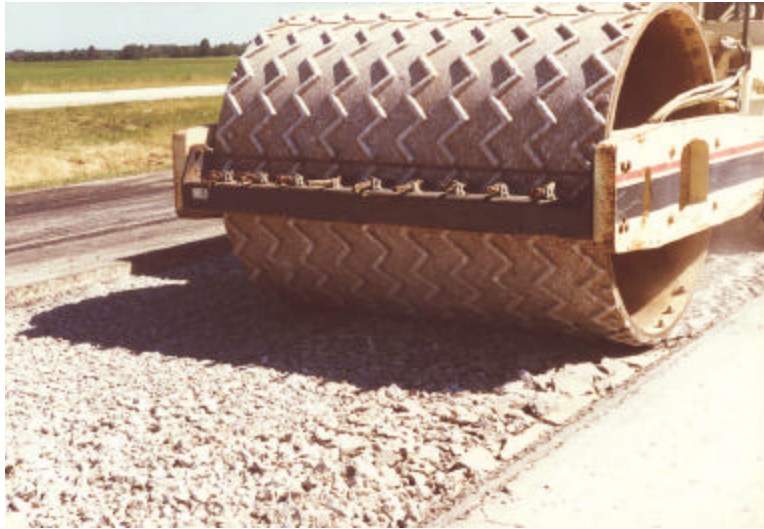
Figure 21. Z-Grid Roller, Longitudinally Attached (I-57 1996).
