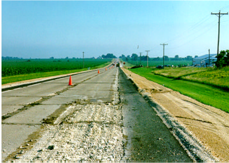
Figure 9. Preconstruction Condition Background, Rubblizing Foreground (IL 38 1994).
