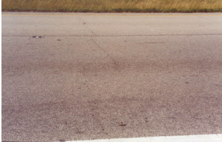
Figure 24. Rubblize and 8" Overlay in 1998 (I-57 1996).
