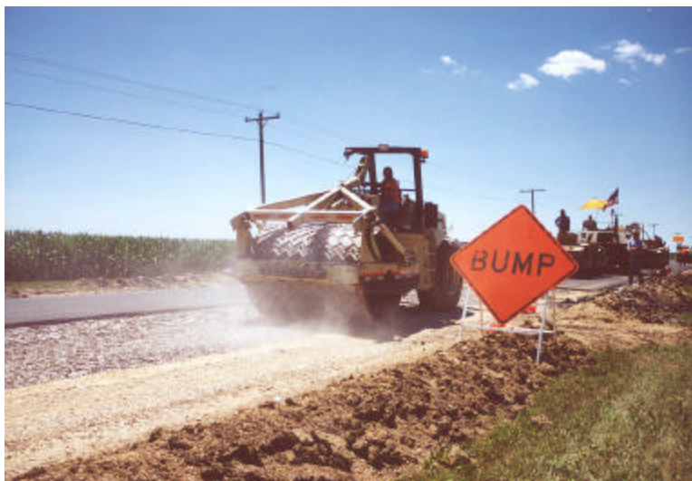
Figure 4. Z-Pattern Steel Grid Roller.
