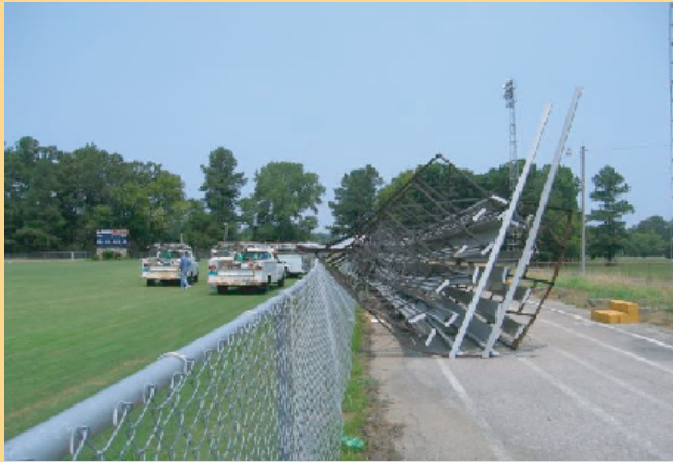
Overturned bleachers at Cherokee High School (Colbert Co.), July 19, 2006
