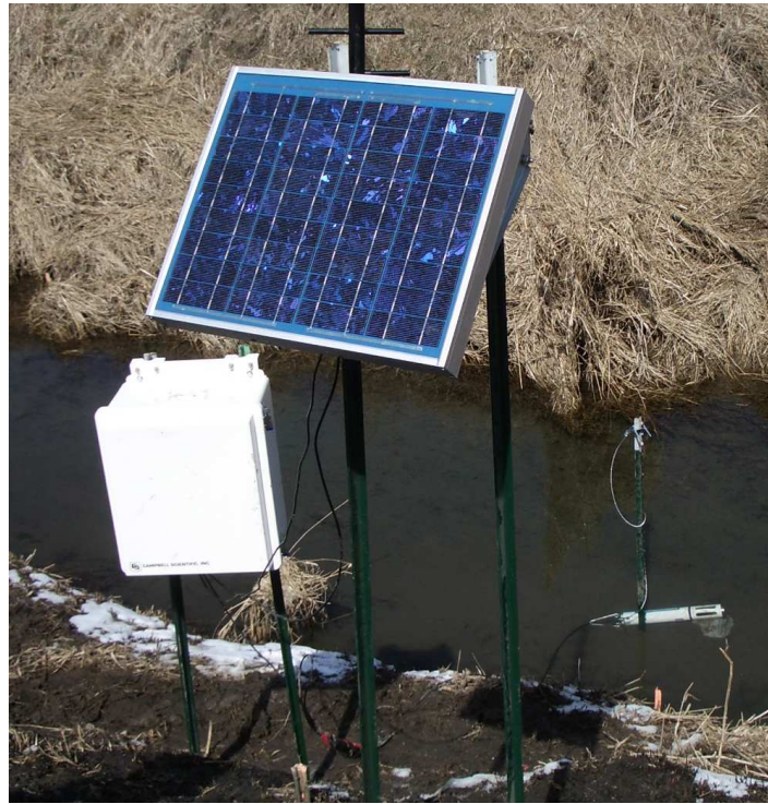
Figure 4. Water quality node installed in Clear Creek, Iowa.
