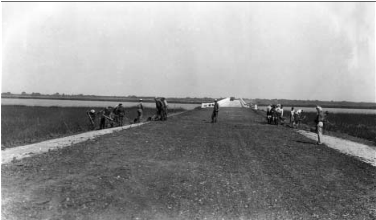
FIGURE 14. CCC enrollees work on South Channel Bridge approach, October 1938
