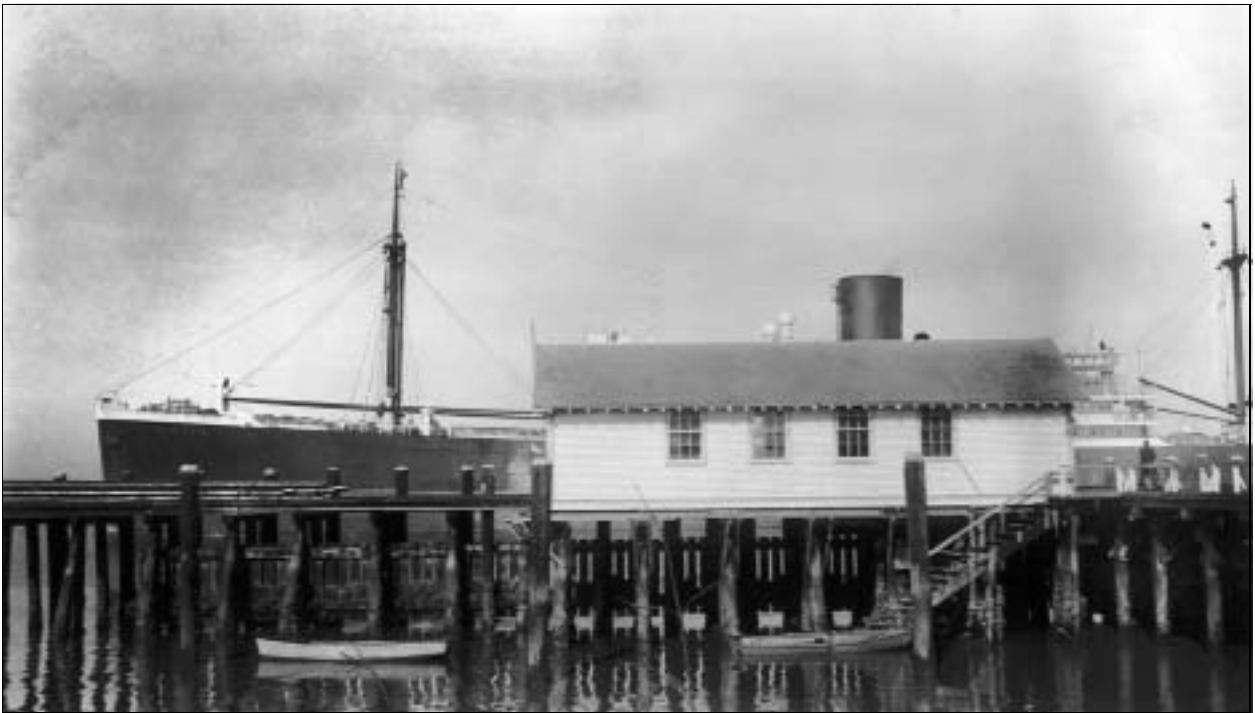
FIGURE 24. NPS wharf on North Channel at old quarantine station, 1938
