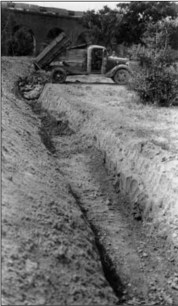
FIGURE 12. Truck dumps moat dirt into parade ground trench, June 1935
