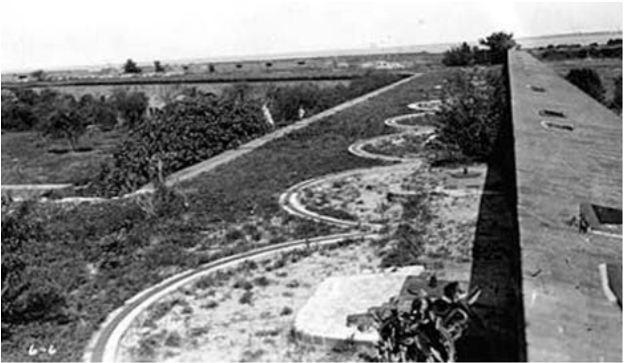
FIGURE 9. View of moat, looking toward the fort, before restoration work, HABS 2158 photo, c. 1930
