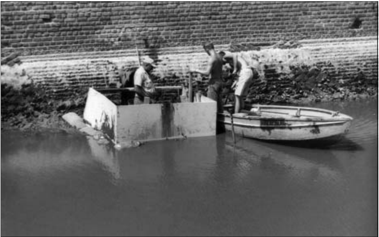
FIGURE 27. Moat maintenance after changing from salt to fresh water, August 1963
