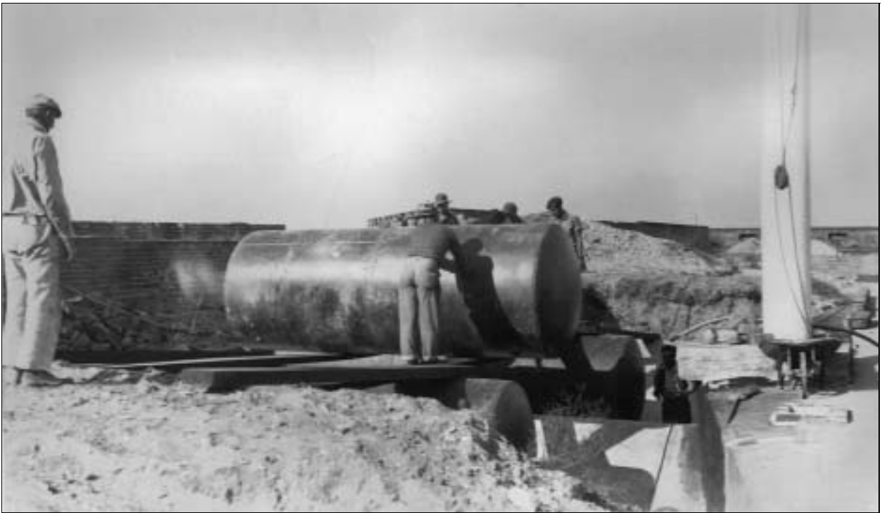
FIGURE 13. PWA installs domestic water tank supply on fort terreplein, November 1935
