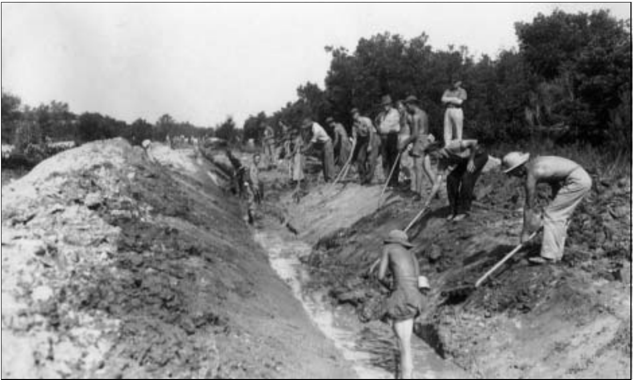
FIGURE 11. CCC enrollees excavate a ditch at Fort Pulaski, May 1936
