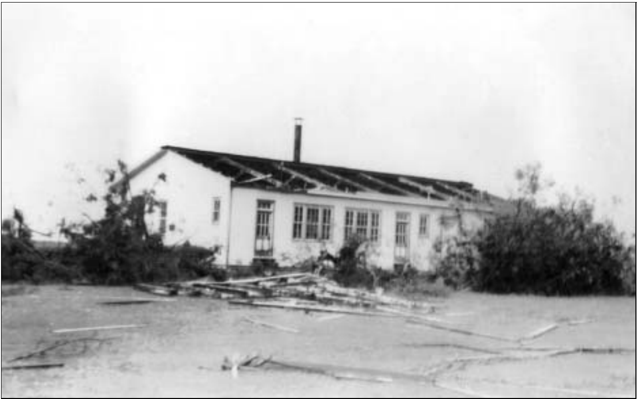
FIGURE 28. Utility building used by CCC after hurricane damage, August 1940
