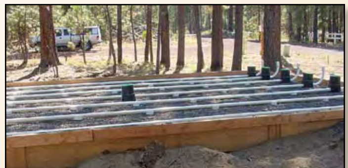
Septic system being installed near La Pine, Oregon.
