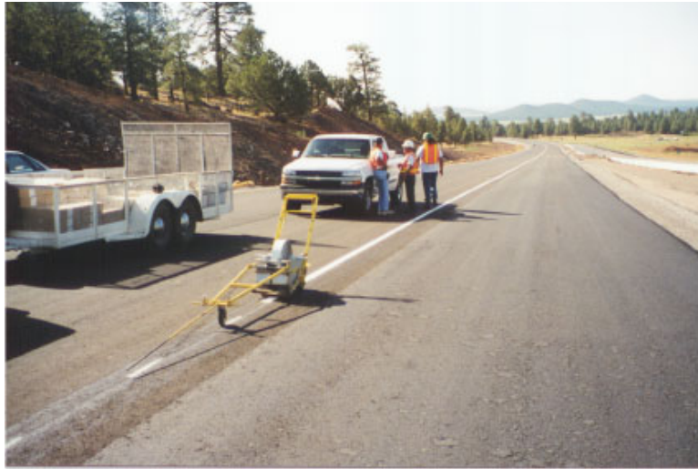
Figure 13: Installation of 3M Tape During US 180 Roadway Construction
