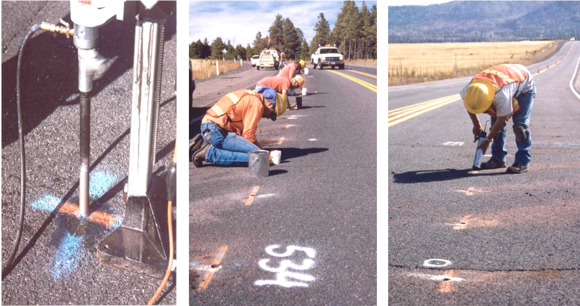
Figure 8: Magnet Installation on US 180: 1998-99
