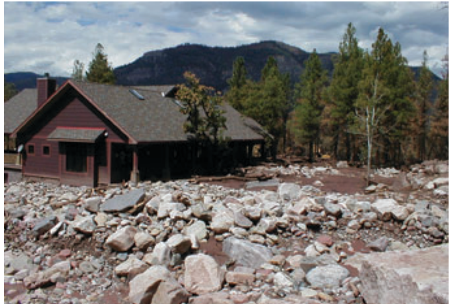
Figure 1. Mudslides occurred on August 4, 2002, after precipitation fell in the burned area of the Missionary Ridge Fire.
