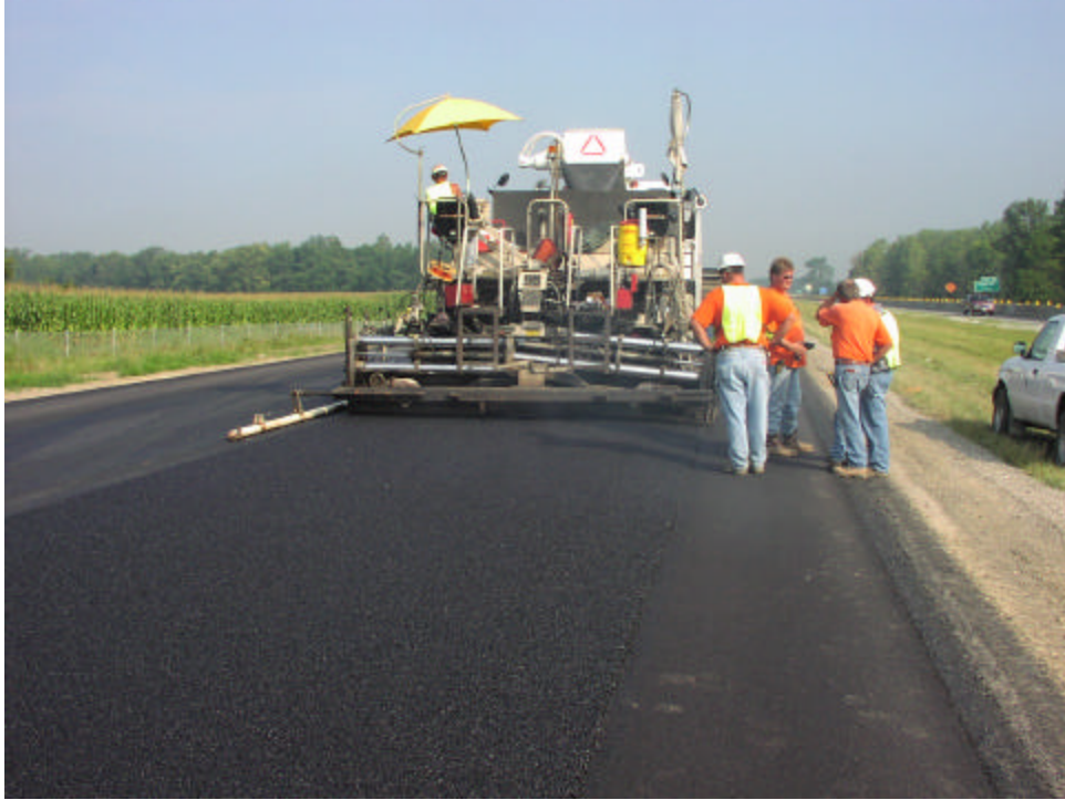
Figure 3. Paver Laying PFC on I74
