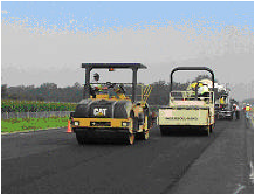
Figure 4. Roller Train Used on I74
