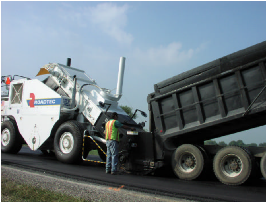
Figure 2. Material Transfer Device Used on I74
