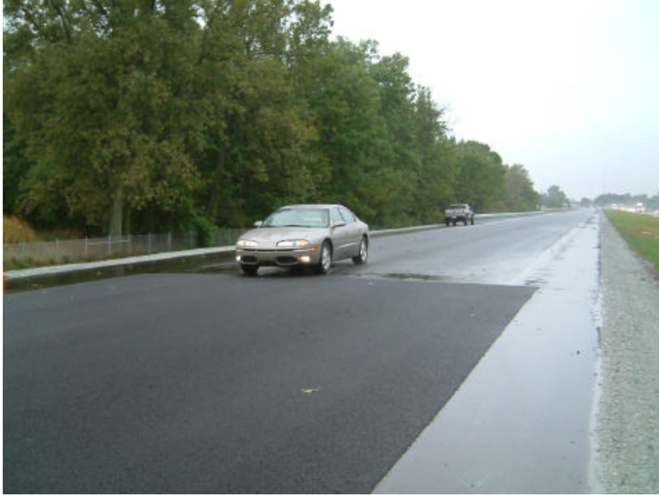
Figure 11. PFC (Left Foreground) vs. SMA (Right Background) during Light Rain
