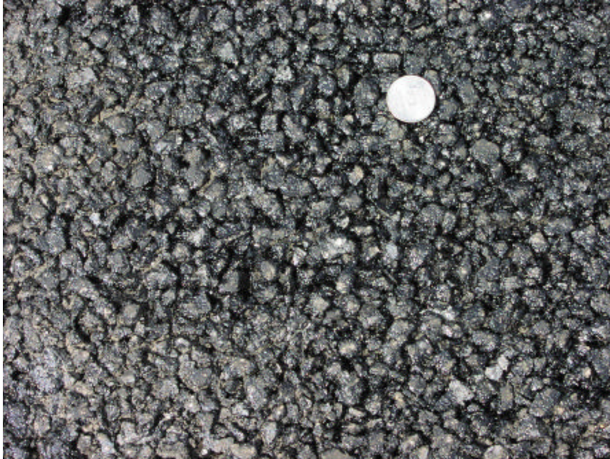
Figure 5. PFC Surface Texture
