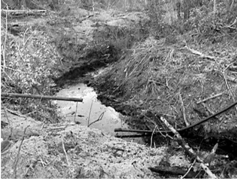
Fallen tree breaks pipeline at James Bayou.
