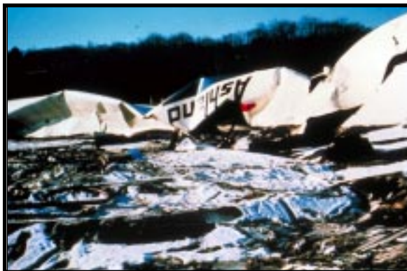
Remains of collapsed four million gallon storage tank.
