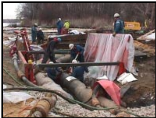
Workers repair a pipeline following an oil spill.
