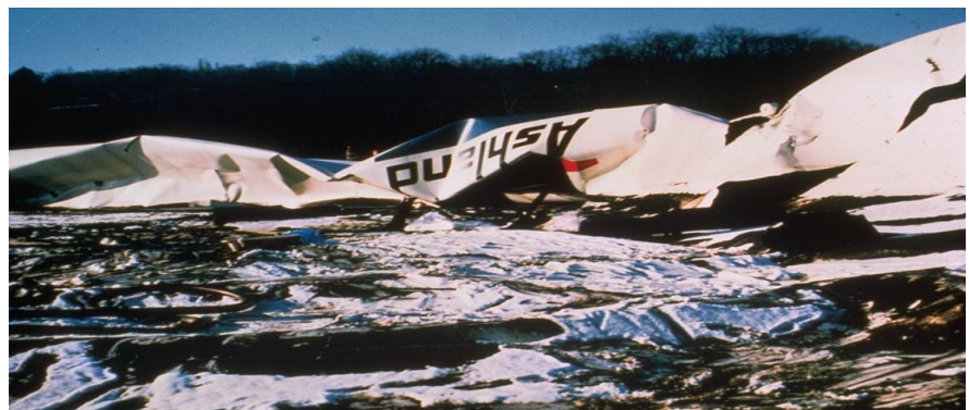
Remains of the collapsed diesel fuel storage tank following the 1988 Ashland spill
