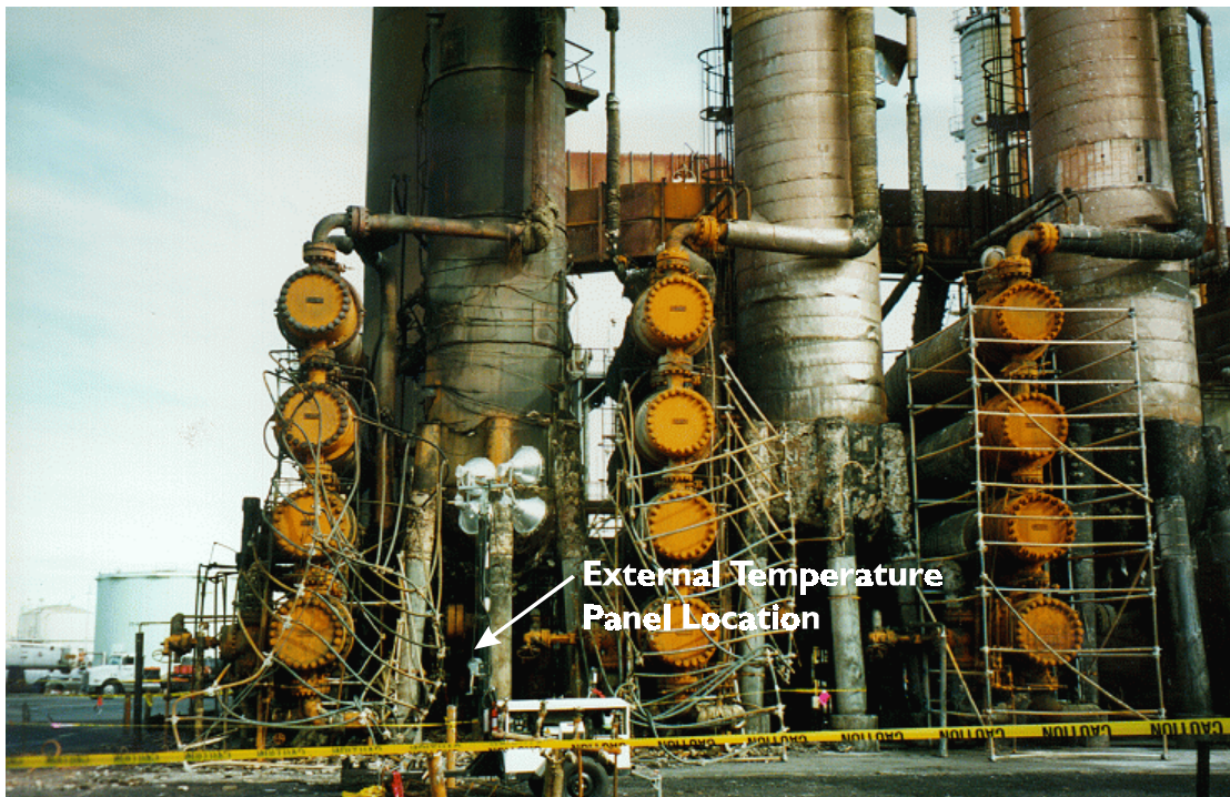
Figure 11 Field Panel Location
