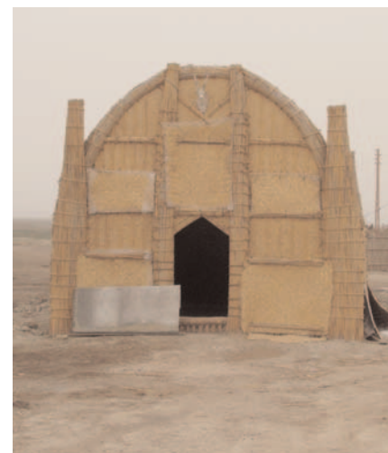
(above and left) The mudhif , a barrel, vaulted, reed structure is indigenous to the marshlands of Iraq.
