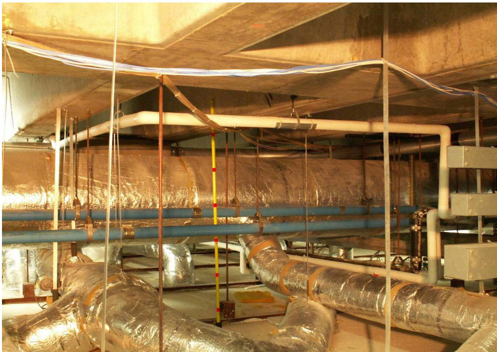
Photo B-2 Interstitial Service Zone Showing HVAC mains in S-3 subzone and branch ducts in S-4 subzone
