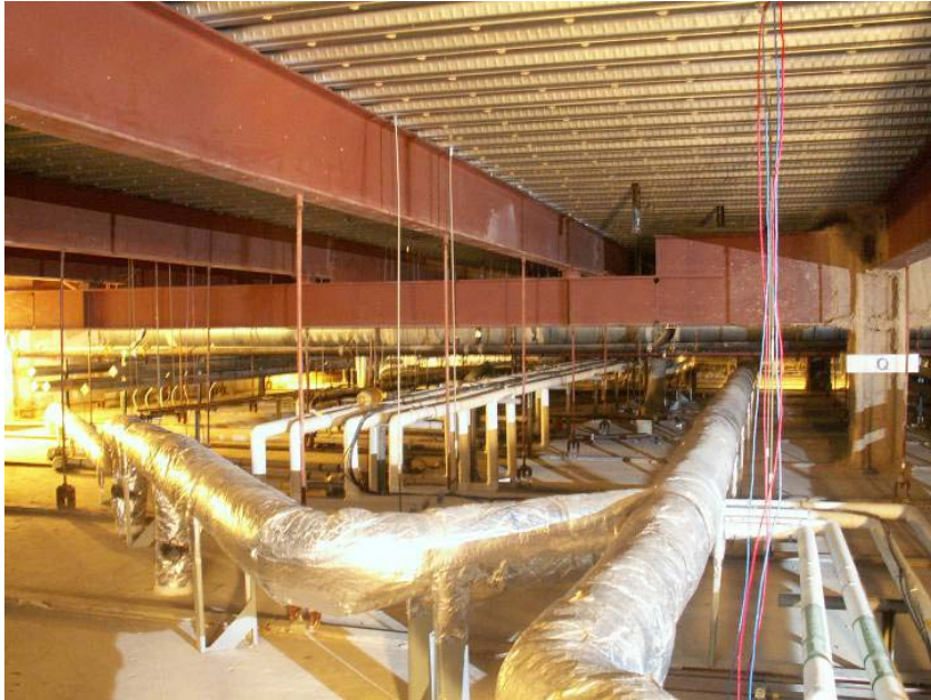
Photo A-5 Interstitial Service Zone Showing typical distribution subzones and channels
