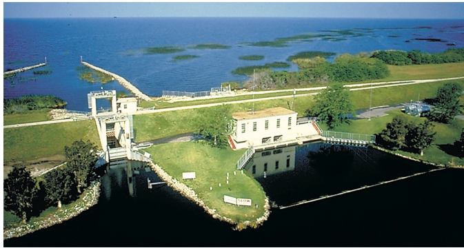
Hoover dike (center) was built with digging spoils obtained from a navigable channel (foreground). Lake Okeechobee is at the top of photo.
