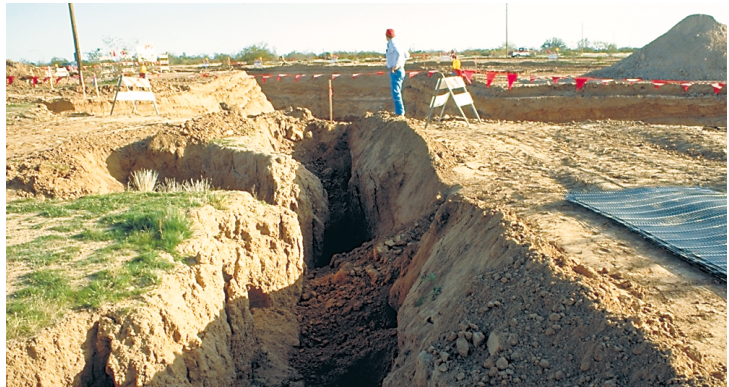
Part of this fissure south of Apache Junction has been trenched and backfilled for a land bridge.
