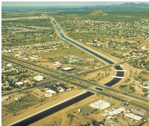
A section of the Central Arizona Project passes through Apache Junction.
