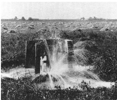
This free-flowing artesian well was capped to prevent waste (1910).
