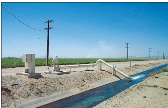
Ground water is withdrawn to dewater the root zone in some agricultural areas.
