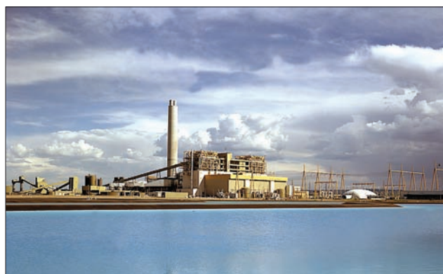
Coronado Thermoelectric Powerplant near St. Johns, Arizona. Photograph courtesy of Salt River Project.
