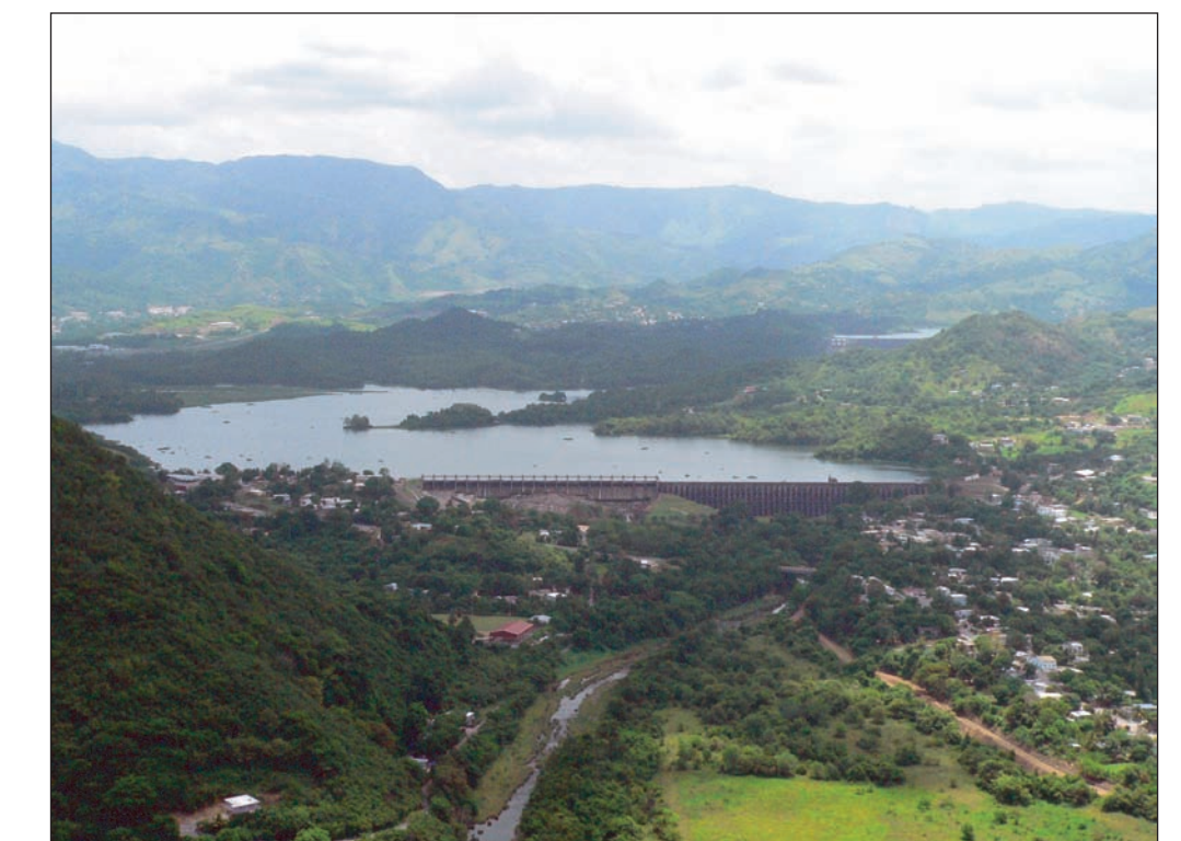
Figure 5. Aerial photograph of the Guayabal Dam and Lago Guayabal looking in the upstream direction. Photograph courtesy of the Puerto Rico Electric Power Authority, taken on May 9, 2006, during a dam-safety inspection helicopter flight.
