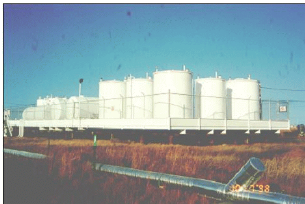
Figure 3-1. Fencing around storage area.
