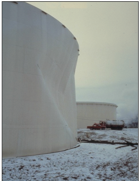
Figure 1-1. Aboveground storage tank in Floreffe, Pennsylvania
