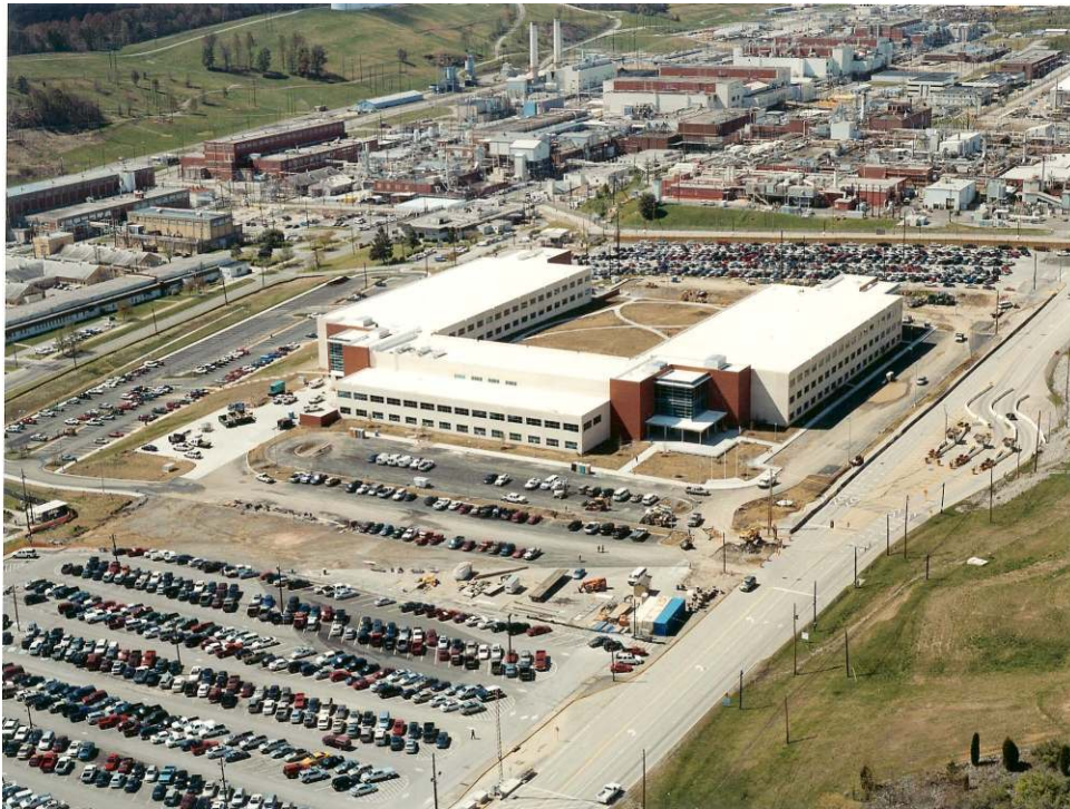
Fig. 7. Y-12 National Security Complex.
