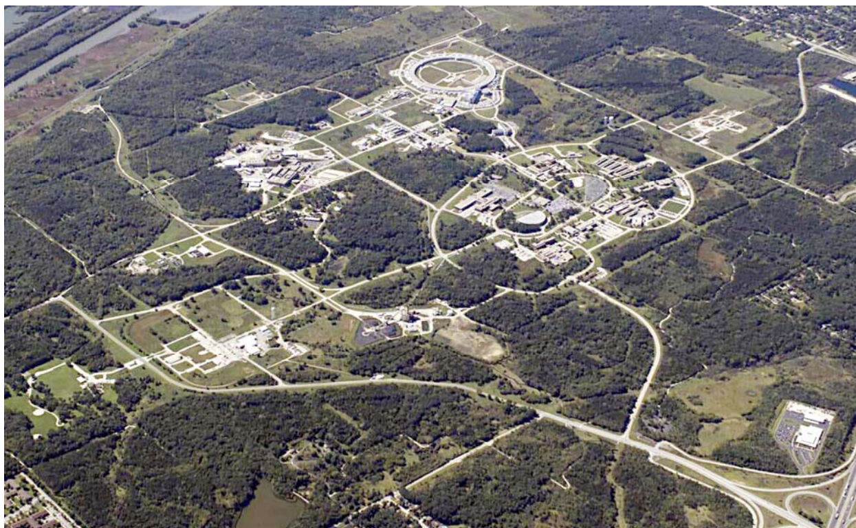
FIGURE B.1 Aerial Image of the Argonne Site
