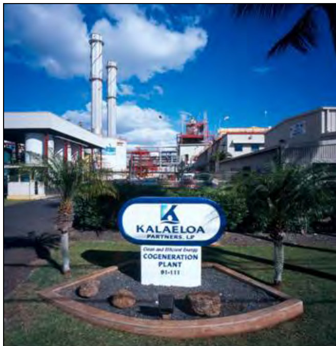
Kalaeloa Partners is one of five companies in the Campbell Industrial Park that utilizes R-O water from the Honouliuli Water Recycling Facility for industrial purposes.
