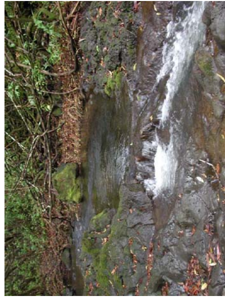
Hau, Hibiscus tiliaceus , encroachment into flood channel of Waiokamilo Stream.
