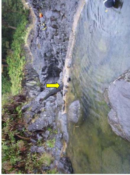
View downstream of diversion pool site gh063r-040208. Black 6" PVC pipe (yellow arrow) in the middle is carrying water downstream. Upper reach Pi'ina'au Stream, Maui, Hawai'i.
