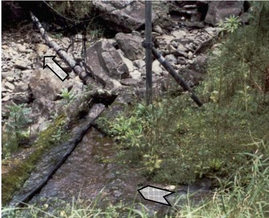
K-30b                      Koolau                      Hauolo Wahine small intake. Concrete-lined ditch.
