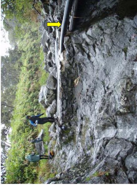
View upstream at next diversion from previous site gh063r-040208. Note 6" black PVC pipe (yellow arrow) on the right which is diverting water from the stream channel and carrying it downstream. Upper reach Pi'ina'au Stream, Maui, Hawai'i.
