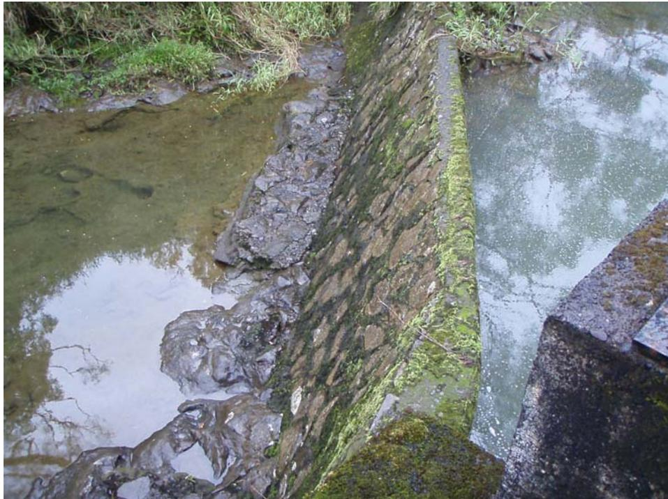
Rock wall dam with metal gate on right on East Wailuanui stream at site sh003\_040308.
