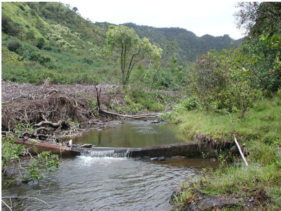
Upstream view of concrete dam on Waiokamilo Stream showing areas where the hau, Hibiscus tiliaceus , are cut back.
