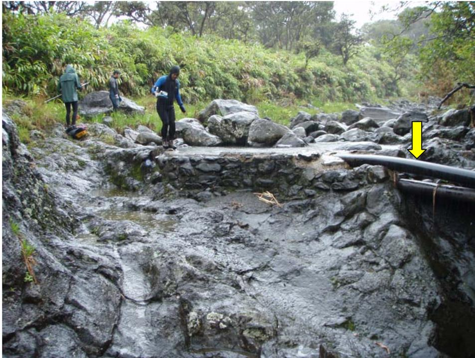
View upstream at next diversion from previous site gh063r-040208. Note 6" black PVC pipe (yellow arrow) on the right which is diverting water from the stream channel and carrying it downstream. Upper reach Pi'ina'au Stream, Maui, Hawai'i.
