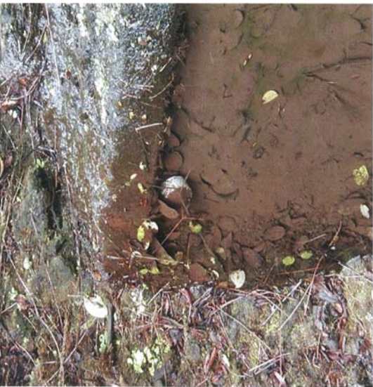
The same 4-inch pipe after the cap was installed.
