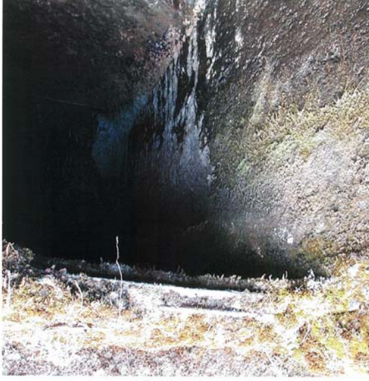
Number 12 intake window sealed with concrete.
