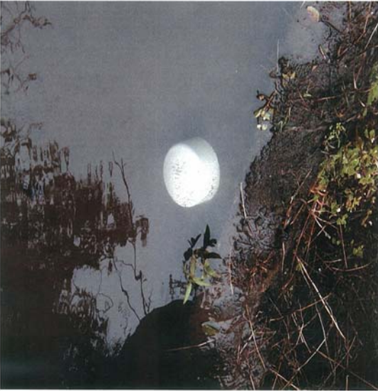
The same 4-inch pipe after cap was installed.
