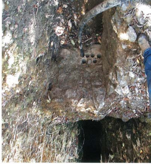
Number 10 intake into the tunnel.
