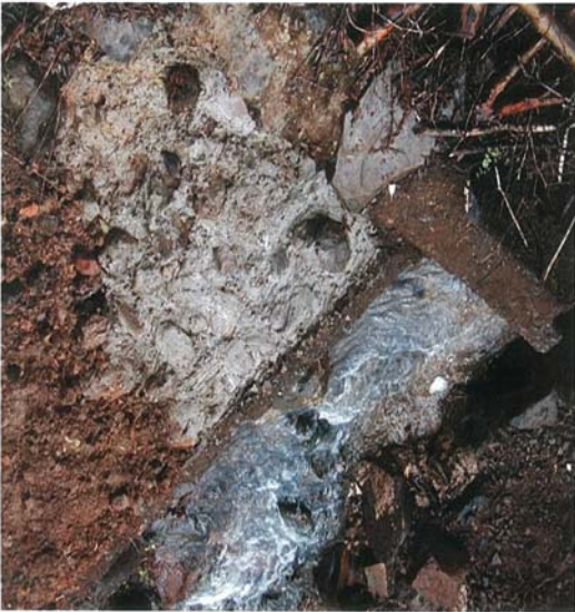
Kualani intake after sealing the pipes and the grate.
