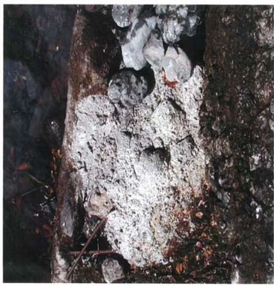
Main Kikokiko intake after it's sealed with rocks and concrete.
