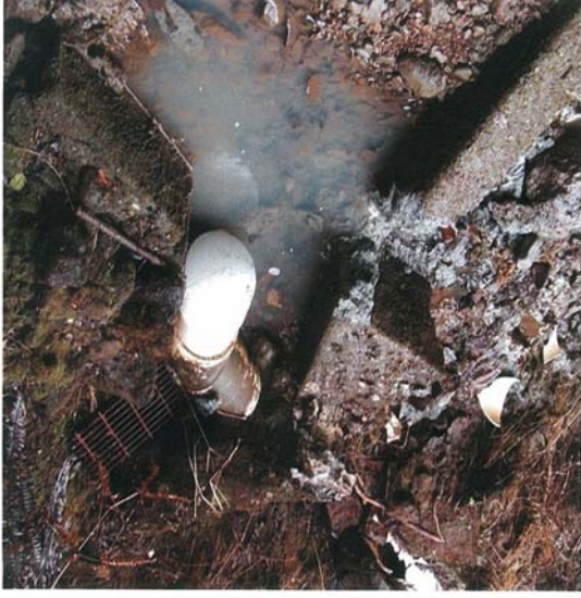
The 8-inch pipe after cap installation and dam breach.
