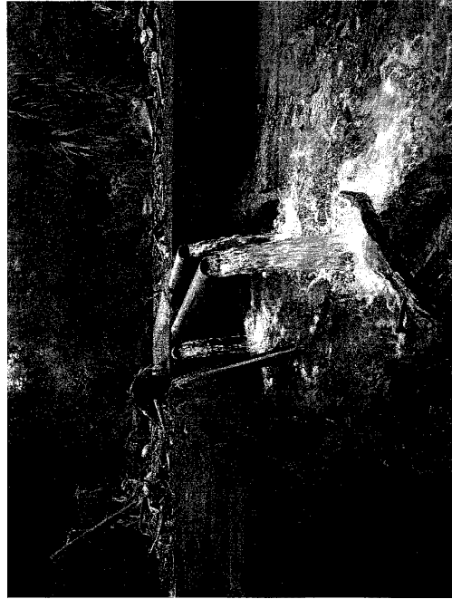
Exhibit "K" – East Maui Irrigation Company Dam on Honopou Stream, with 3 pipes in background allowing water to flow past dam and rest to flow in Haiku Ditch at right.
