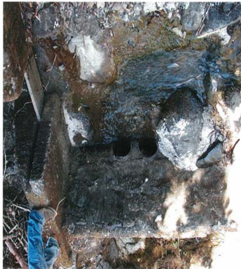
Kualani intake before sealing the pipes and the grate.
