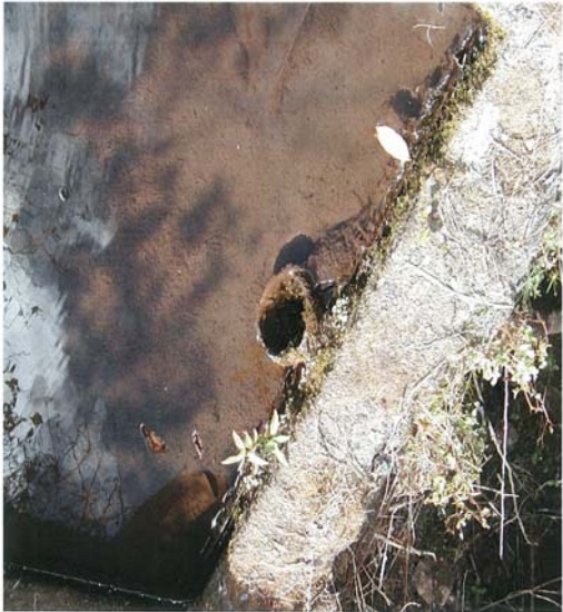
A 4-inch pipe before cap is installed.
