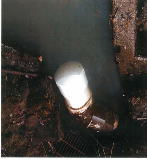
The 8-inch pipe before dam breach.
