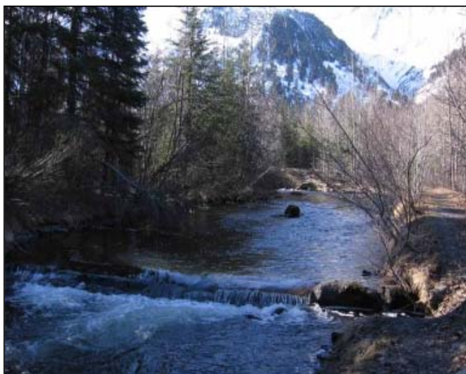
Figure 7. The Structure Reach of Daves Creek, showing the second log weir and the user trail. The culvert is just upstream of the photograph
