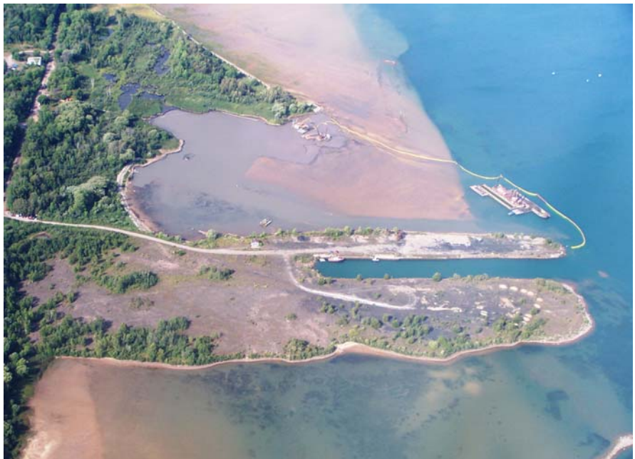
Aerial view of Tannery Bay. The dredging operation platform can be seen on the right.
