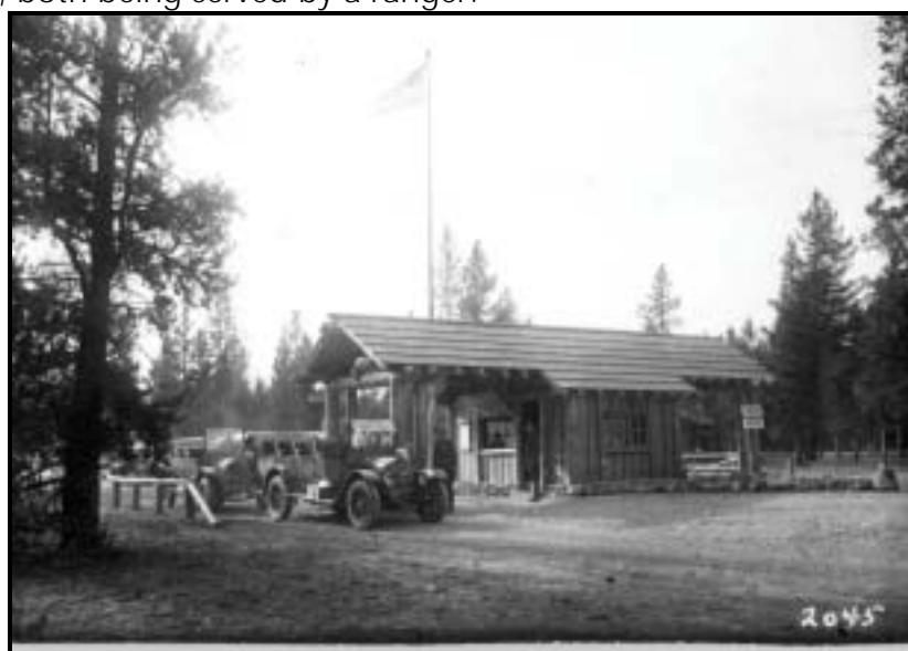
West Entrance, 1932 (the third entrance on this site).
