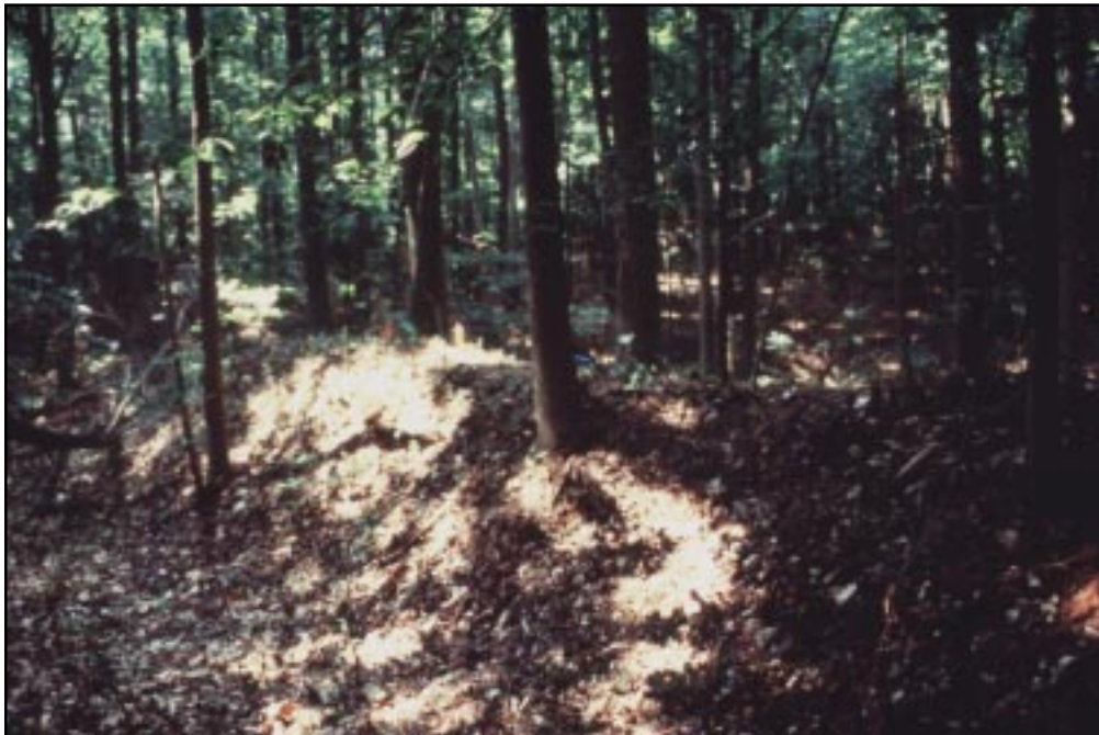
Figure 3.3. Protected earthwork on Main Unit of Petersburg National Battlefield. Forest canopy is closed and forest floor is intact, providing ideal protection. Erosion is nonexistent.
