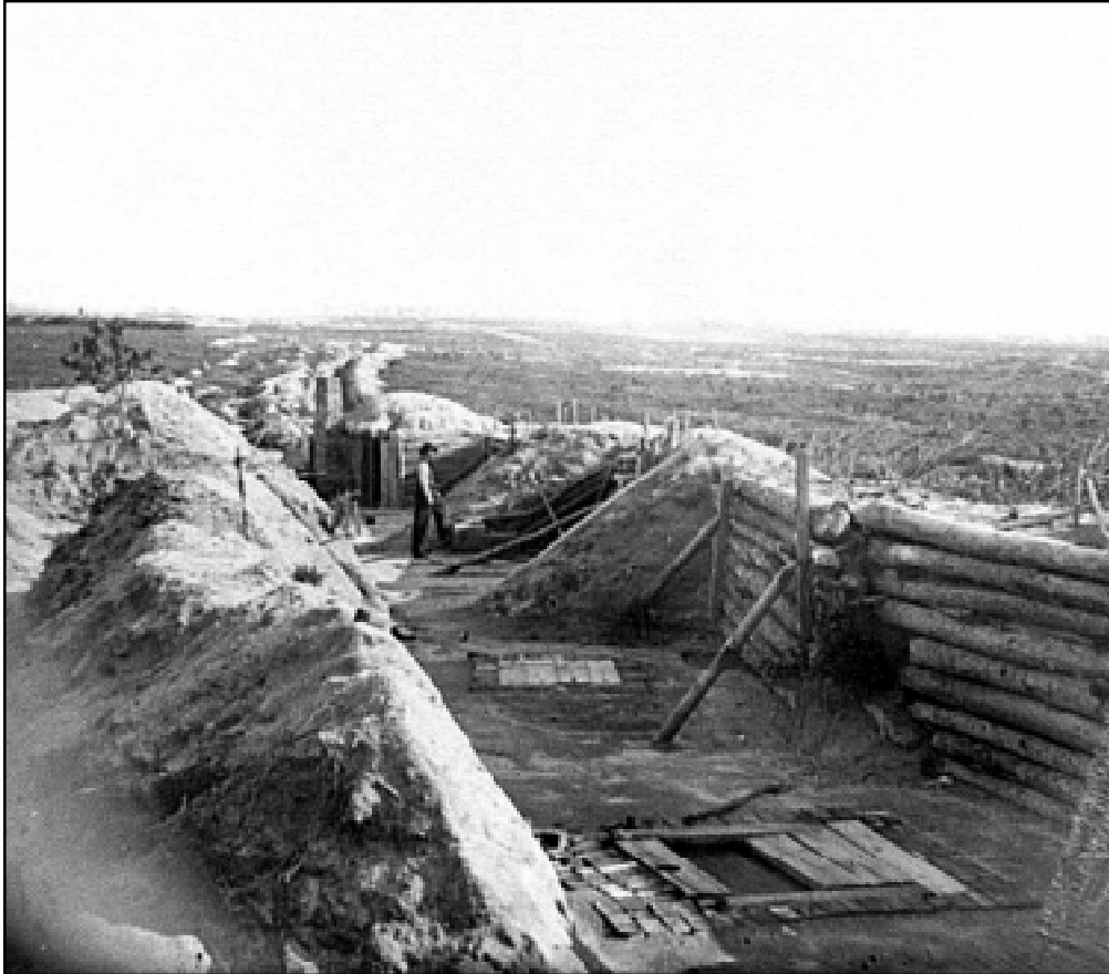
Figure 1.4. This photograph taken in 1865 shows an example of ditch-in-rear construction, using a log revetment, along a federal line near Fort Morton, Petersburg, Virginia.
