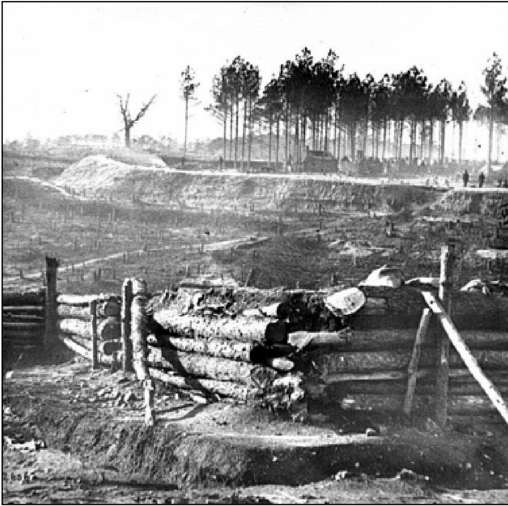
Figure 1.1. This 1864 photograph of federal earthworks near Point of Rocks, Bermuda Hundred, Virginia shows the extensive tree clearing which often accompanied large scale earthworks construction.
