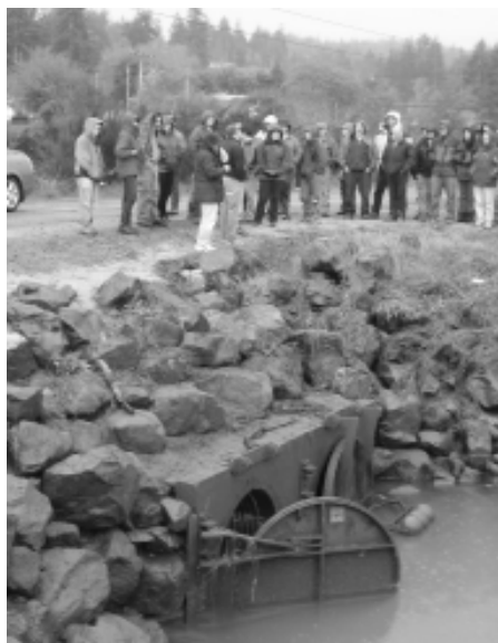
Workshop attendees get a close view of the sidehinge tide gate on Coalbank Slough.
