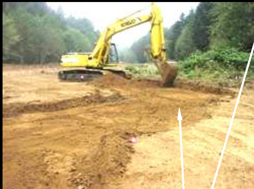
High flow channel under construction
