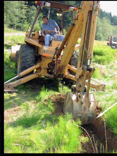
Low flow channel under construction
