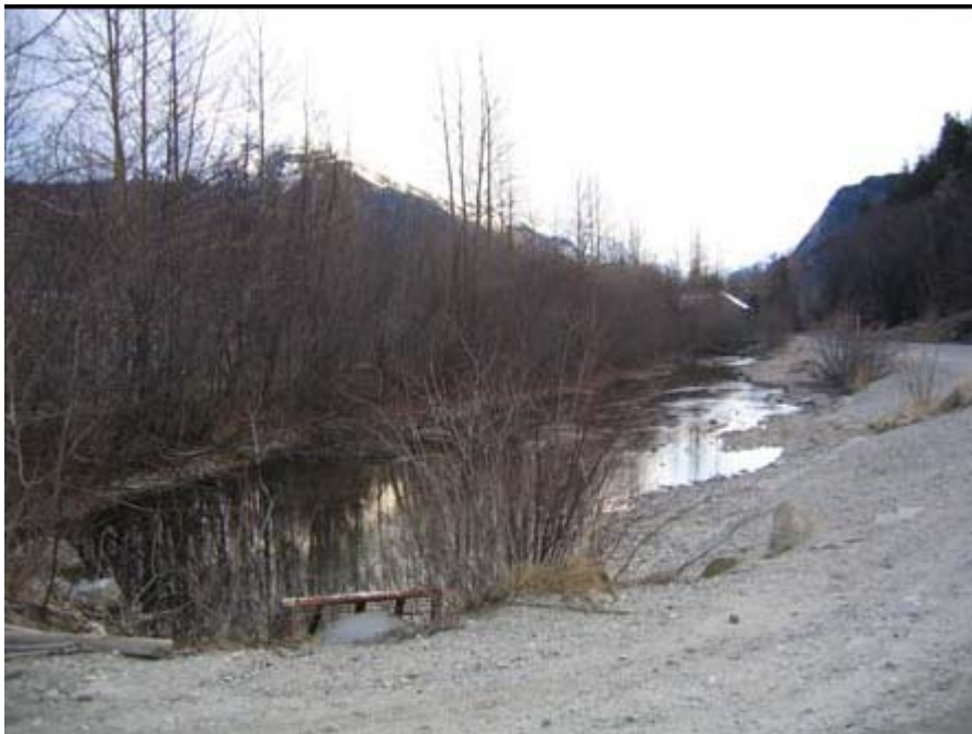
Area of Pullen Creek affected by perched culverts.
