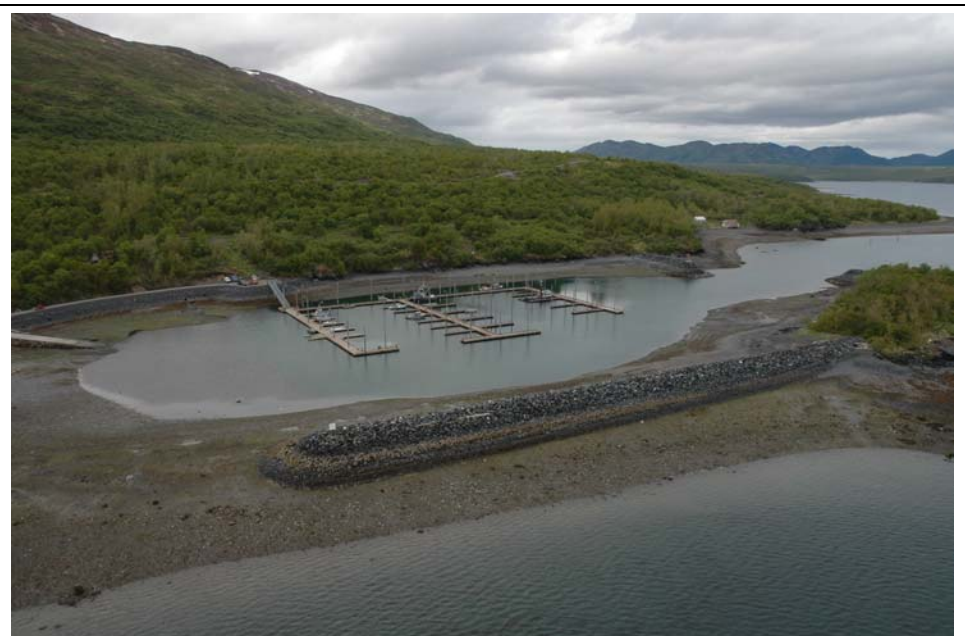
The unit in the foreground includes Forms for breakwater ("Ab") composed of riprap (Materials="Ar").
