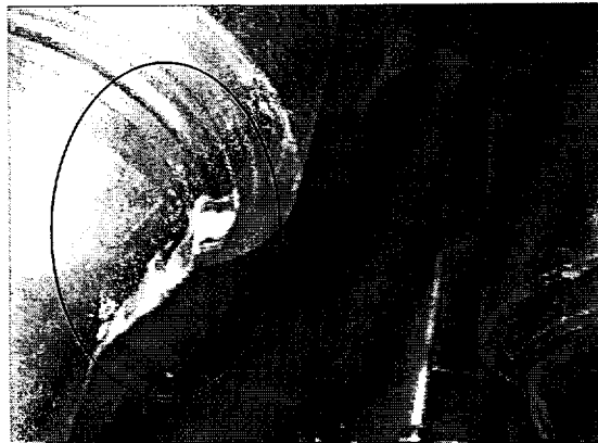
Figure 3. Typical Visual Indication of Leakage from Canopy Seal Weld Area
