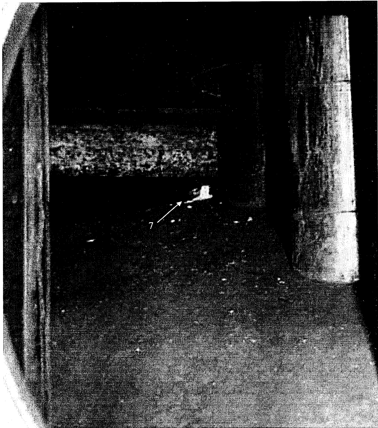
Figure 1 Oconee Unit 1 CRDM Nozzle 7, Top of RV head inspection for Boric acid crystals, 03/31/02
